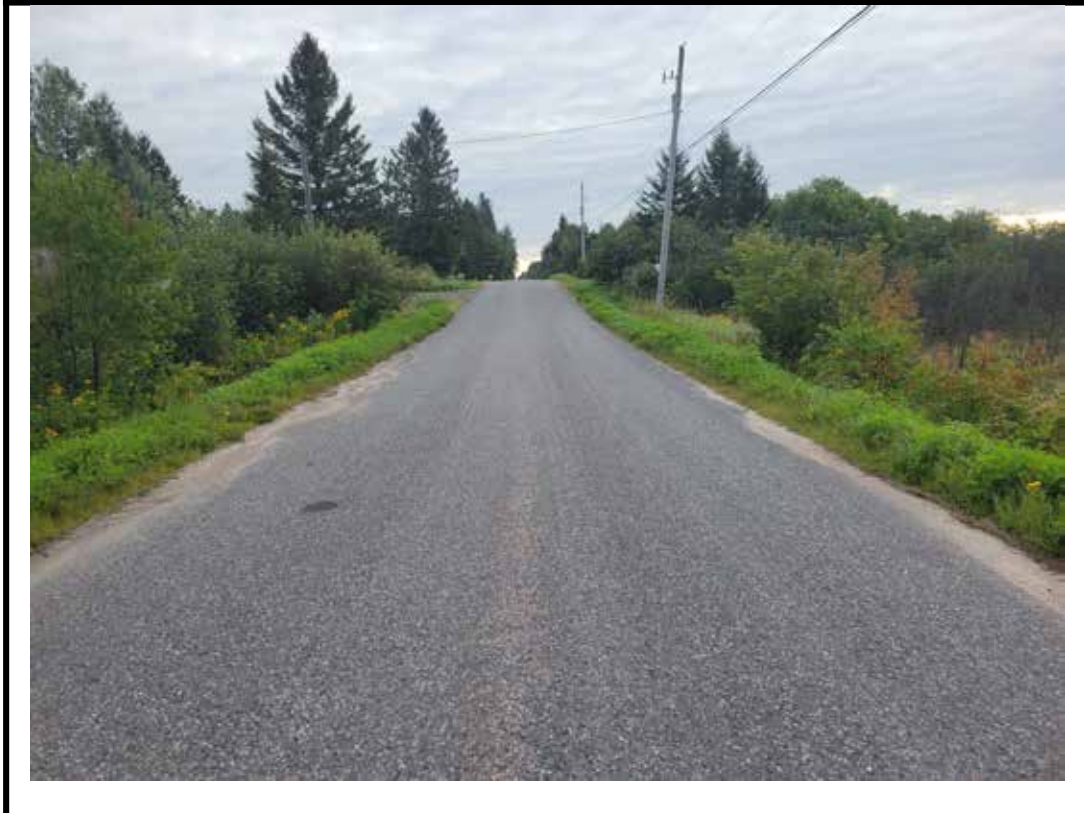
Photo 4 West approach from center of structure
