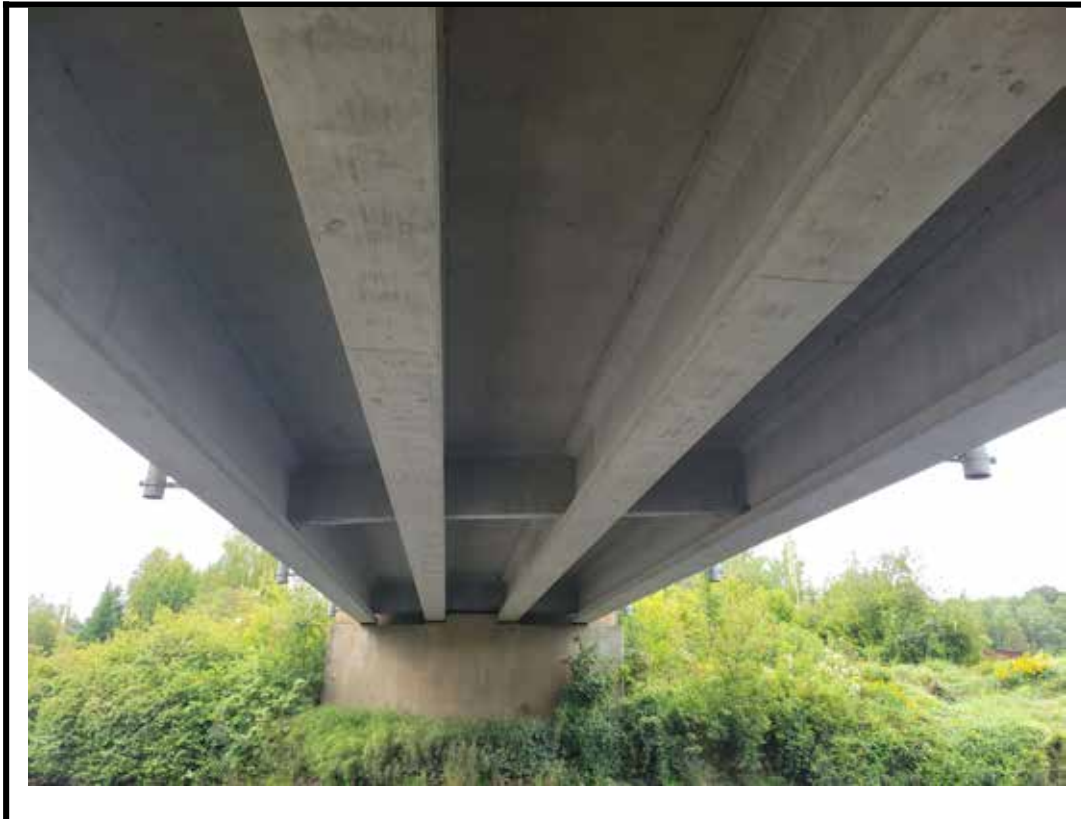
Photo 13 General underside of structure
