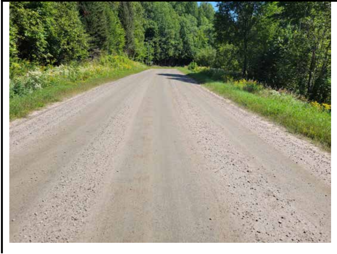
Photo 3 East approach from center of structure
