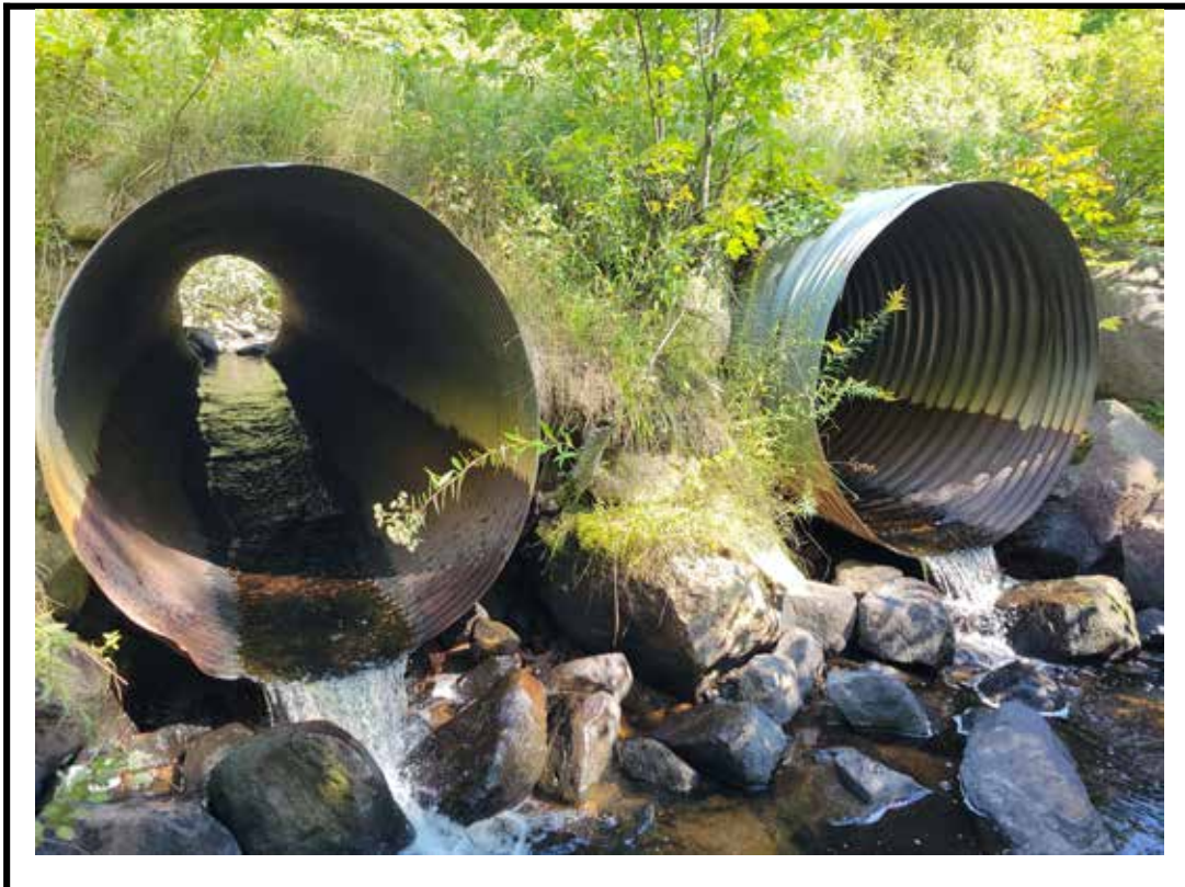
Photo 12 West end of both barrels are perched
