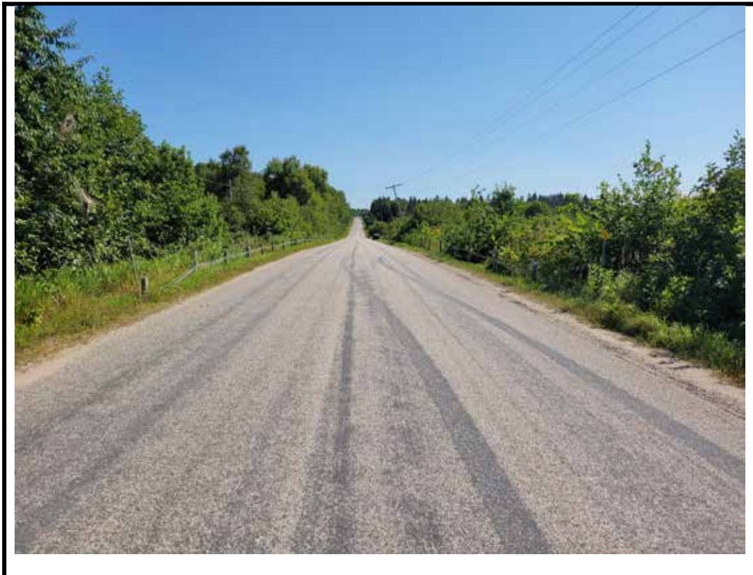
Photo 2 Structure from west approach
