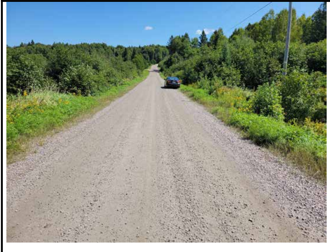
Photo 2 Structure from west approach
