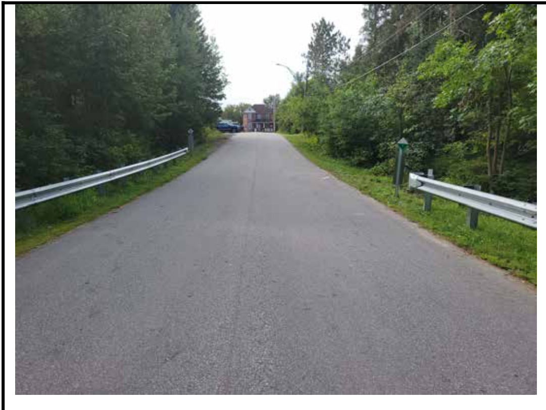
Photo 4 South approach from center of structure
