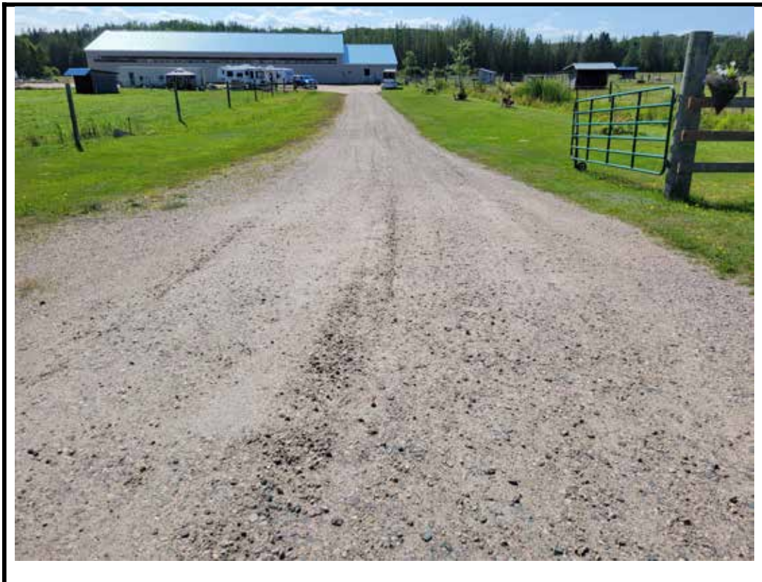
Photo 4 West approach from the center of structure
