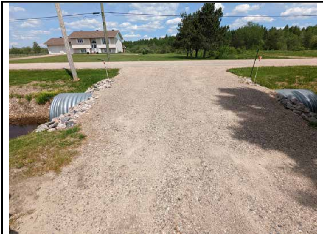
Photo 2 Structure from West approach
