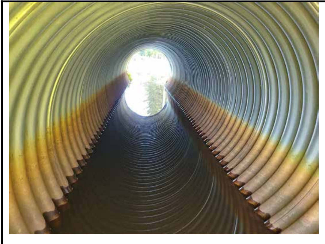
Photo 7 Interior of culvert barrel
