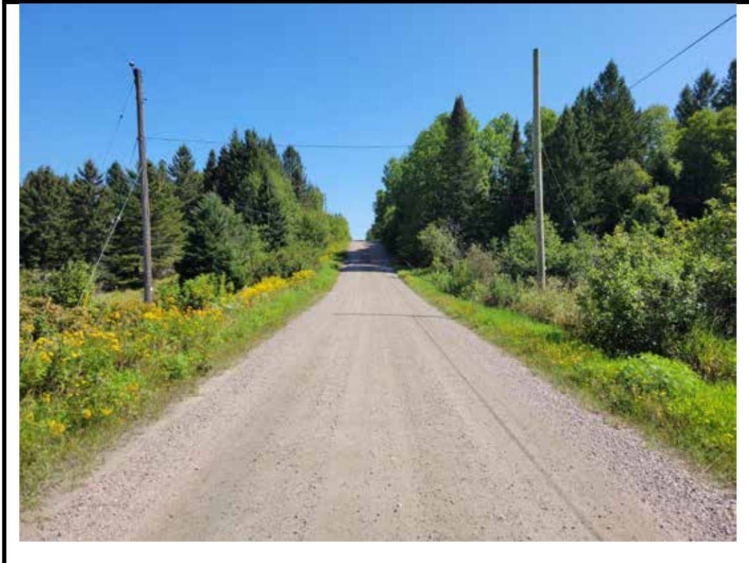
Photo 2 Structure from west approach
