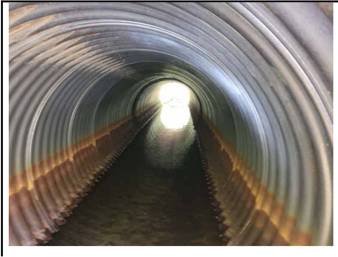
Photo 7 Interior of culvert barrel
