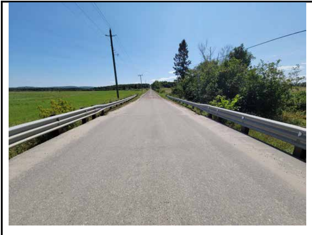
Photo 4 South approach from center of structure
