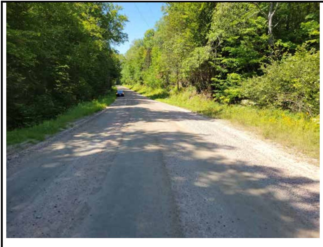
Photo 2 Structure from south approach
