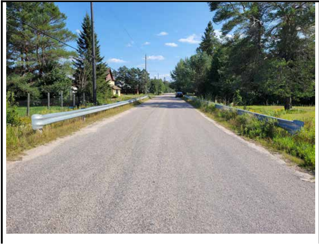
Photo 1 Structure from north approach
