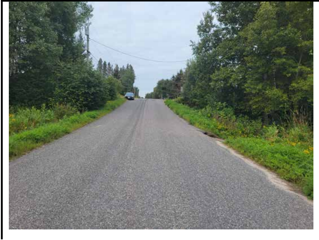
Photo 3 East approach from center of structure
