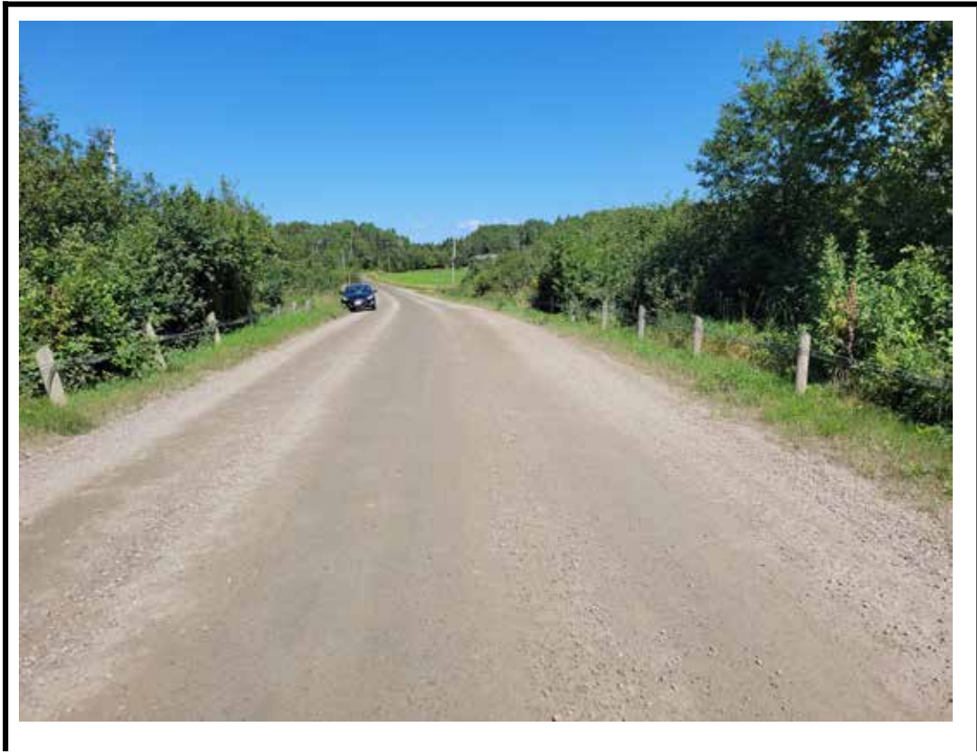
Photo 3 North approach from center of structure
