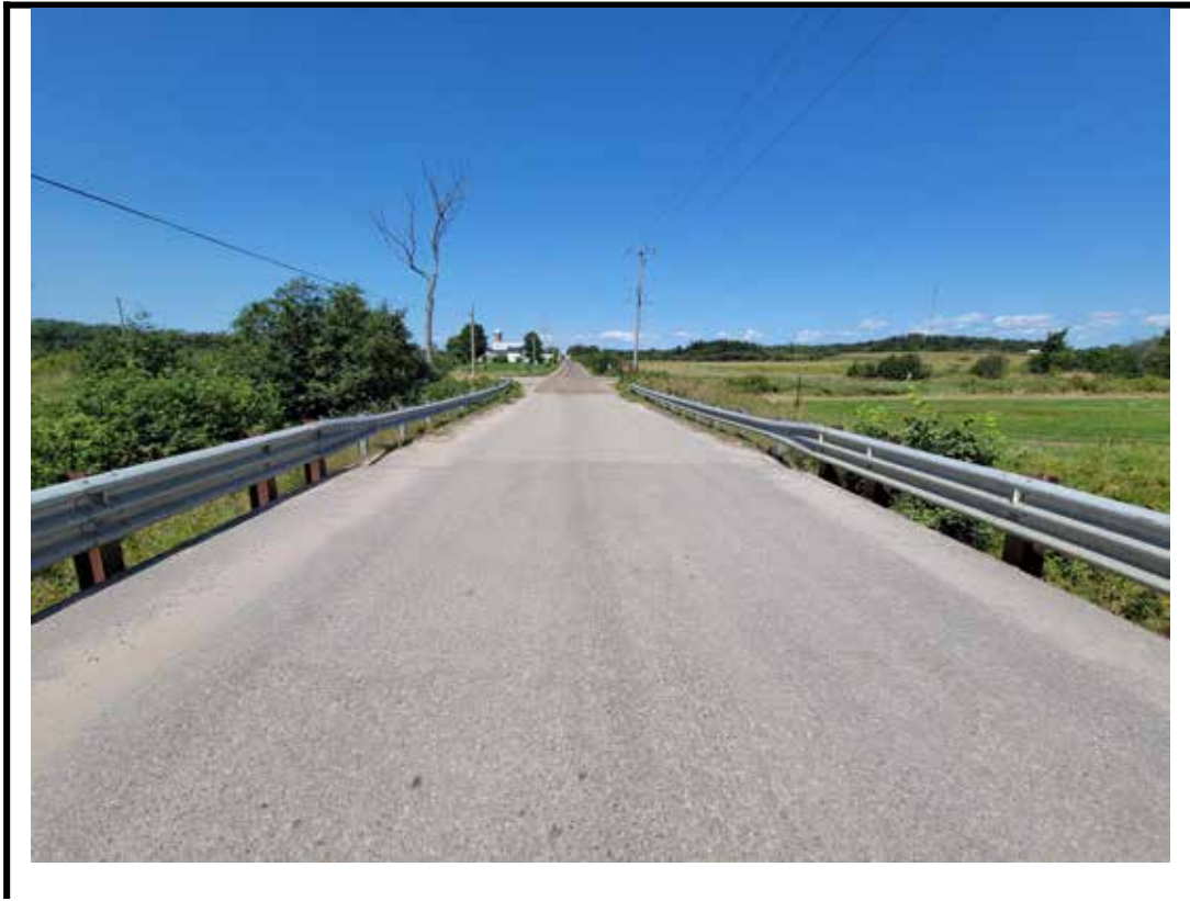
Photo 3 North approach from center of structure
