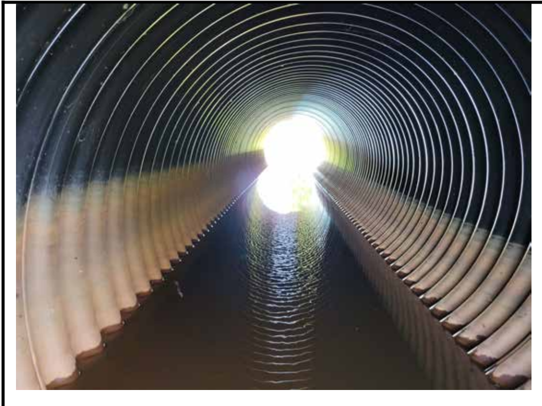
Photo 7 General view of barrel looking south
