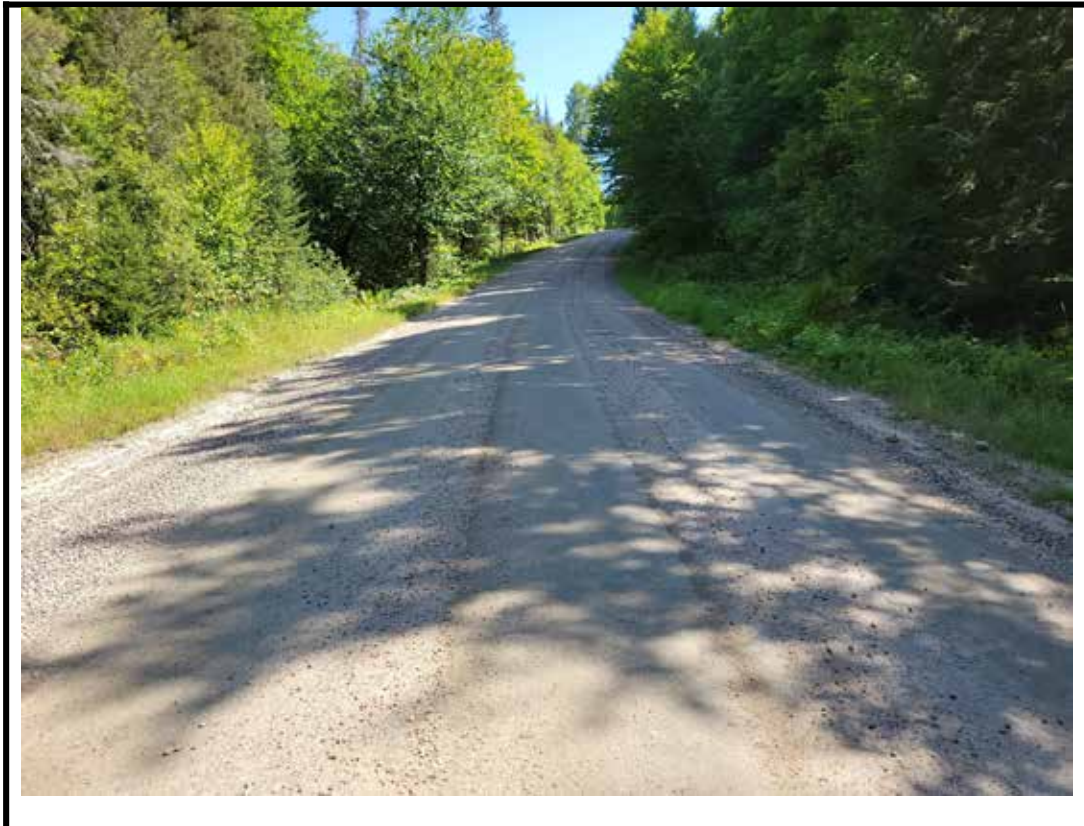
Photo 4 South approach from center of structure
