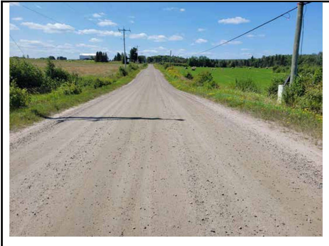
Photo 4 West approach from center of structure
