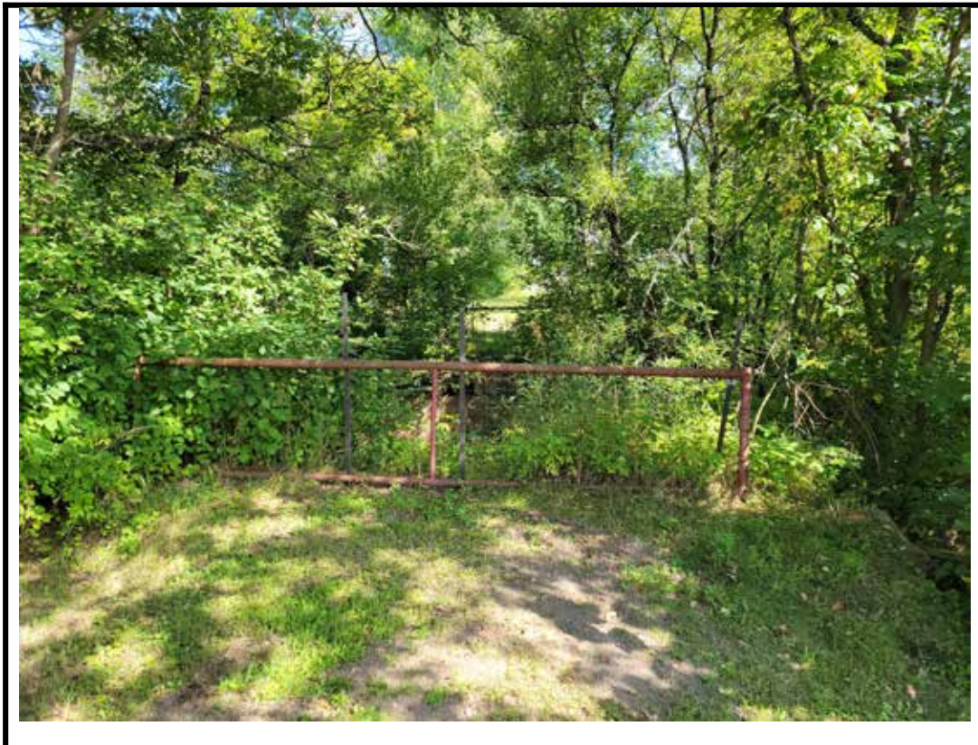
Photo 2 Structure from south approach
