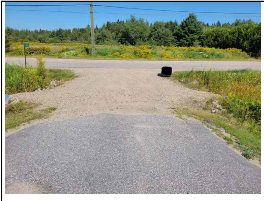
Photo 2 Structure from West approach
