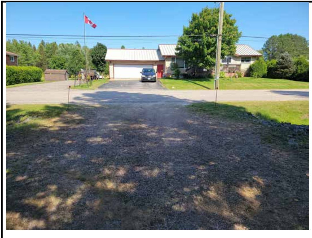
Photo 2 Structure from West approach
