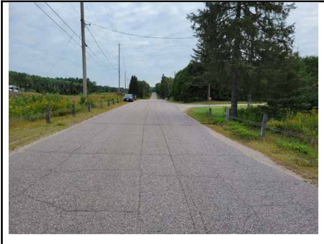
Photo 3 North approach from center of structure
