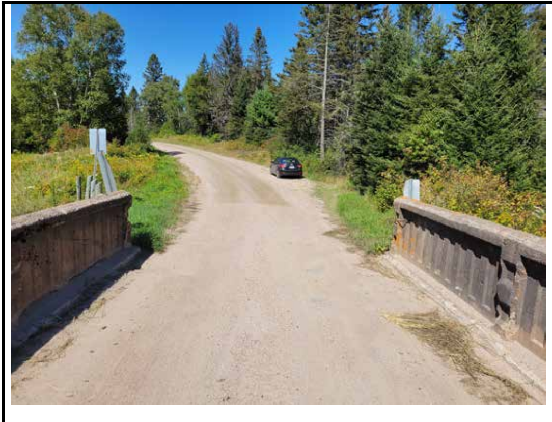
Photo 3 North approach from center of structure
