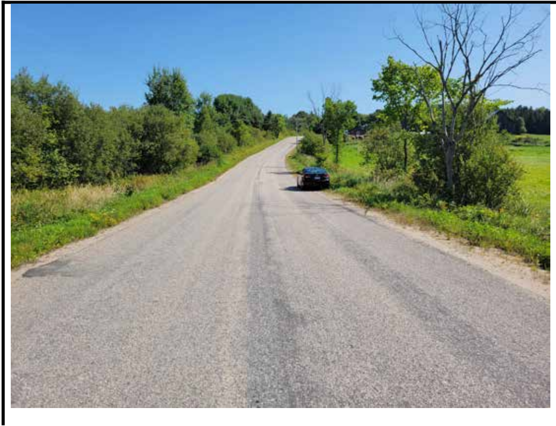
Photo 3 East approach from center of structure
