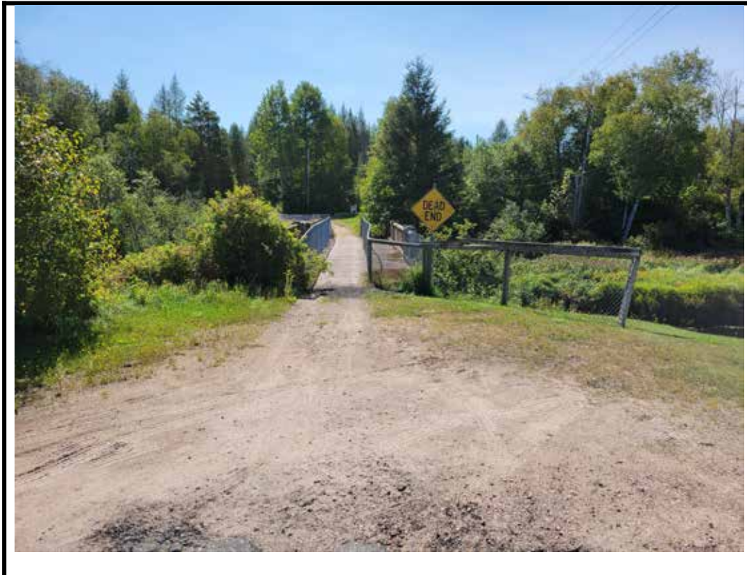
Photo 1 Structure from east approach
