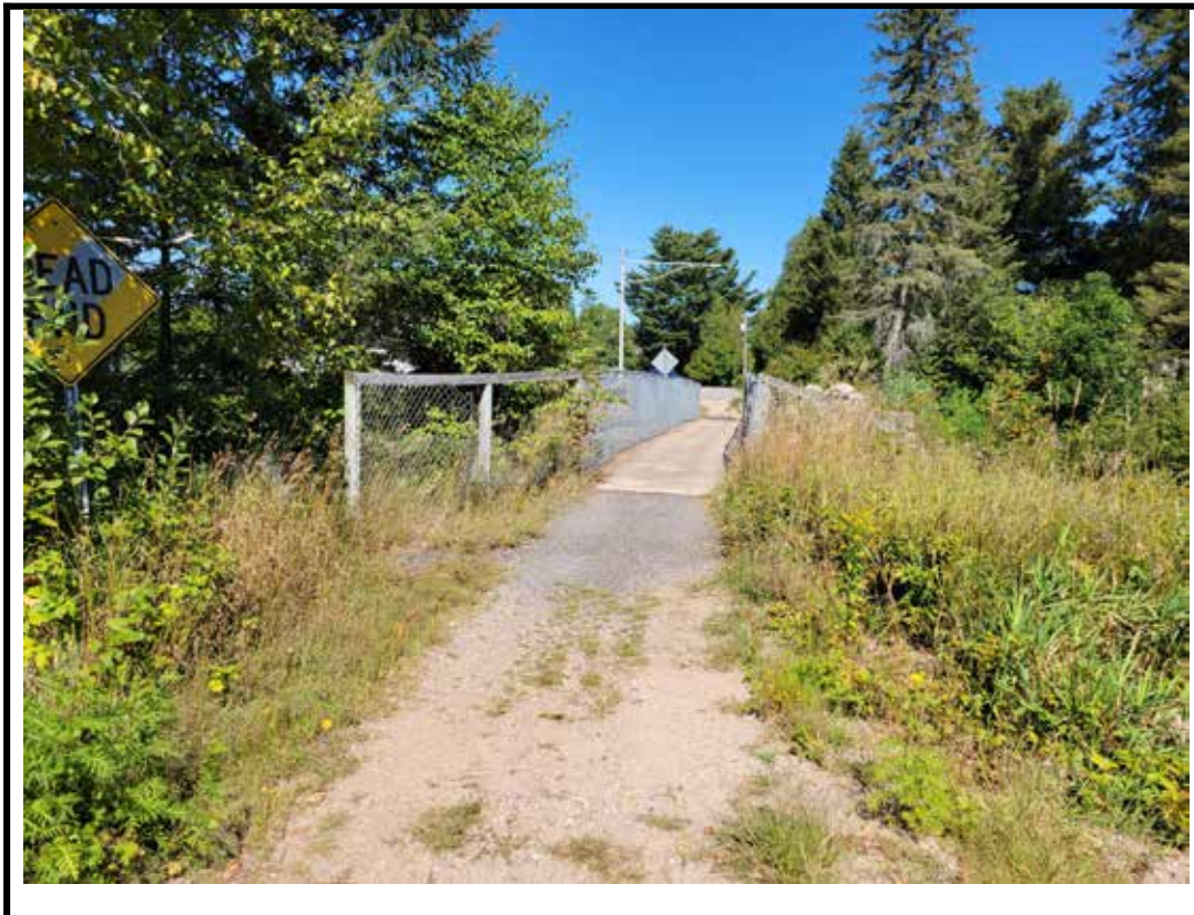
Photo 2 Structure from west approach
