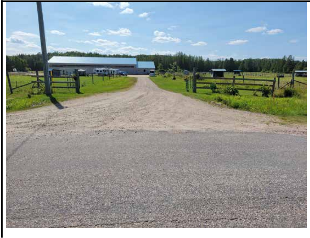
Photo 1 Structure from East approach
