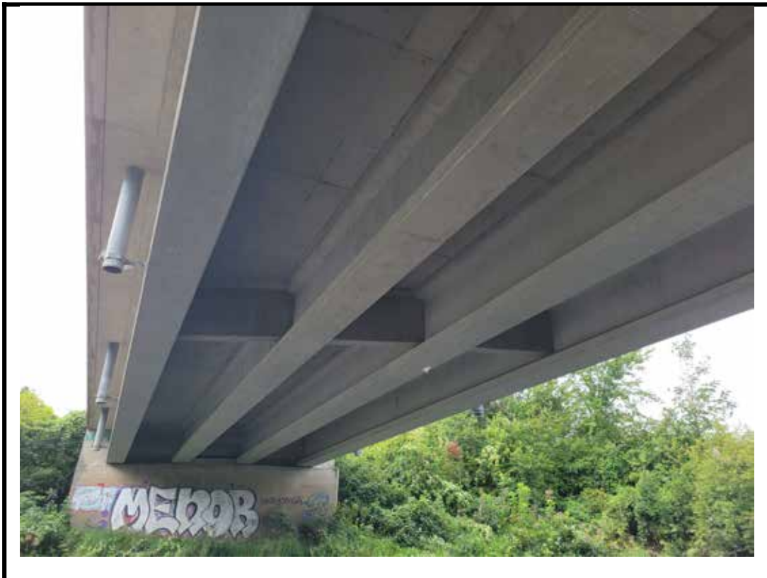
Photo 14 General underside of structure
