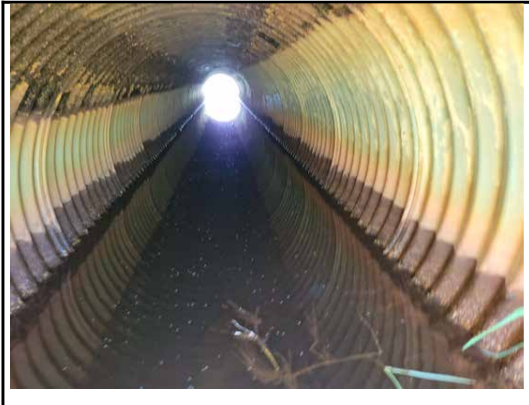
Photo 9 Interior of east culvert barrel
