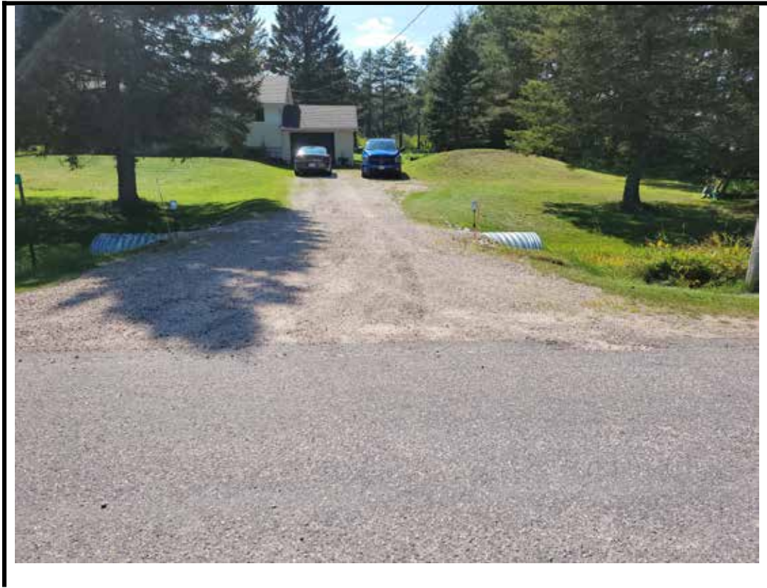
Photo 1 Structure from East approach
