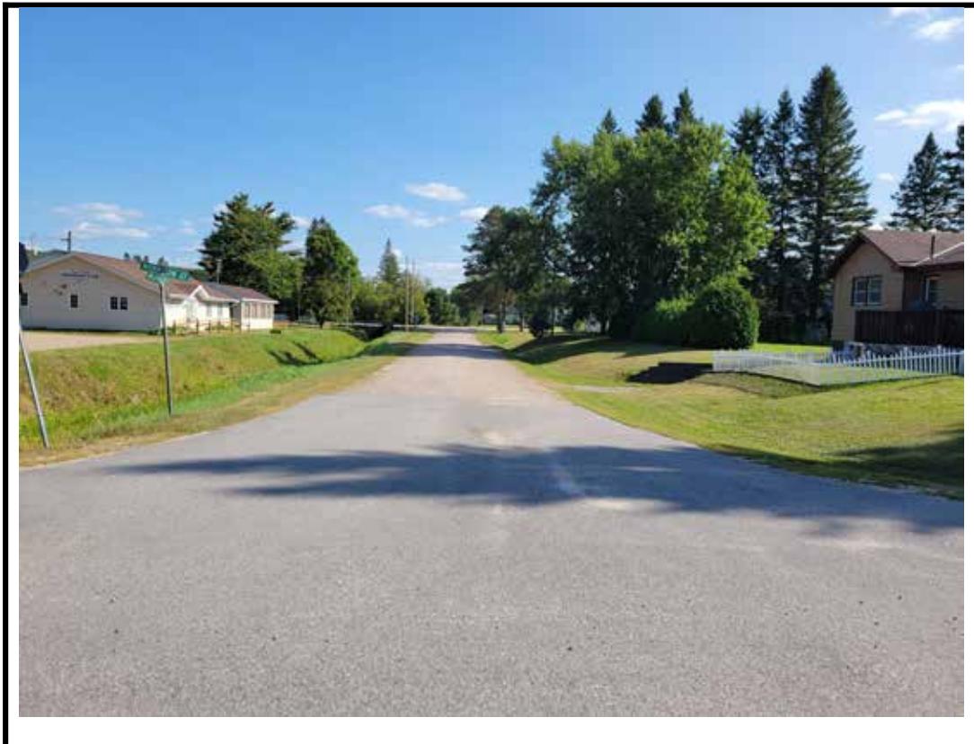
Photo 4 South approach from center of structure
