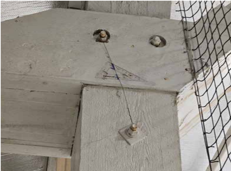
Photograph 9: Representative monitoring between column and adjacent structure
