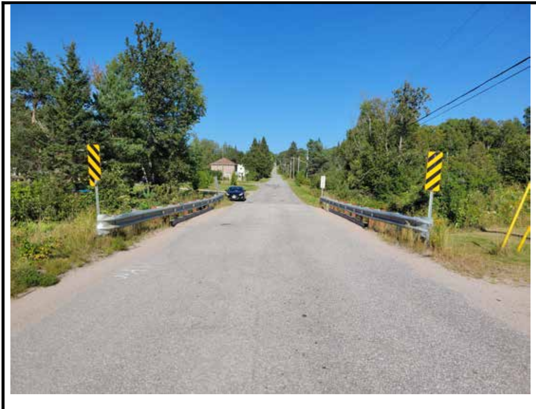
Photo 2 Structure from west approach
