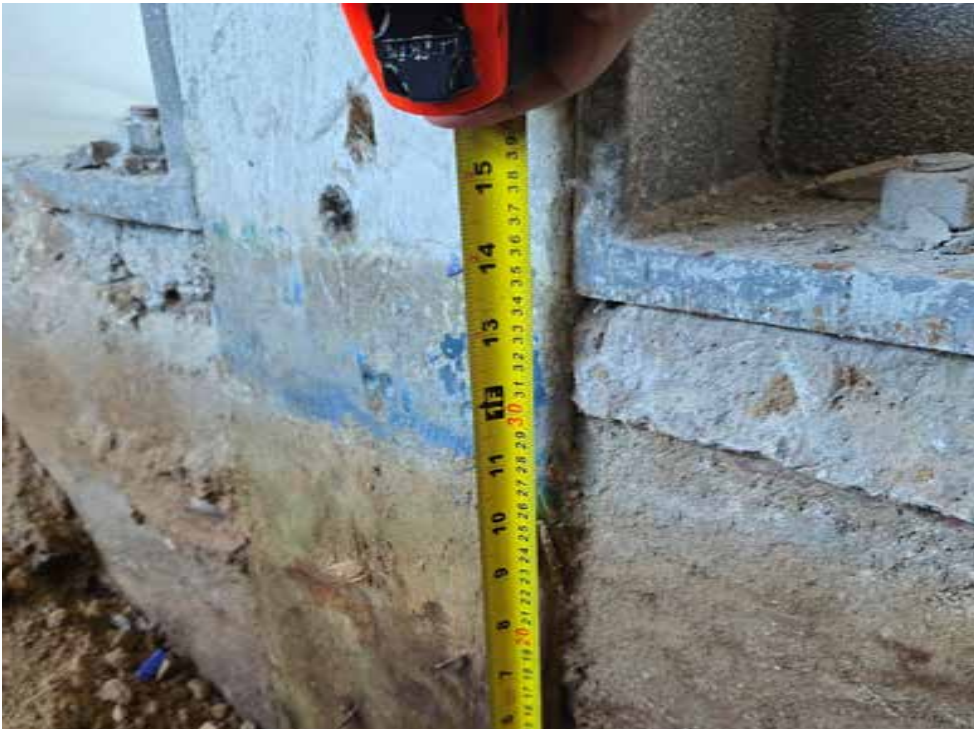
Photograph 4: Retrofit bolted steel plate bearing - interior column
