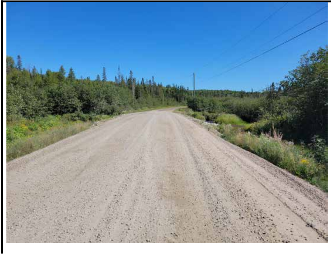
Photo 1 Structure from east approach
