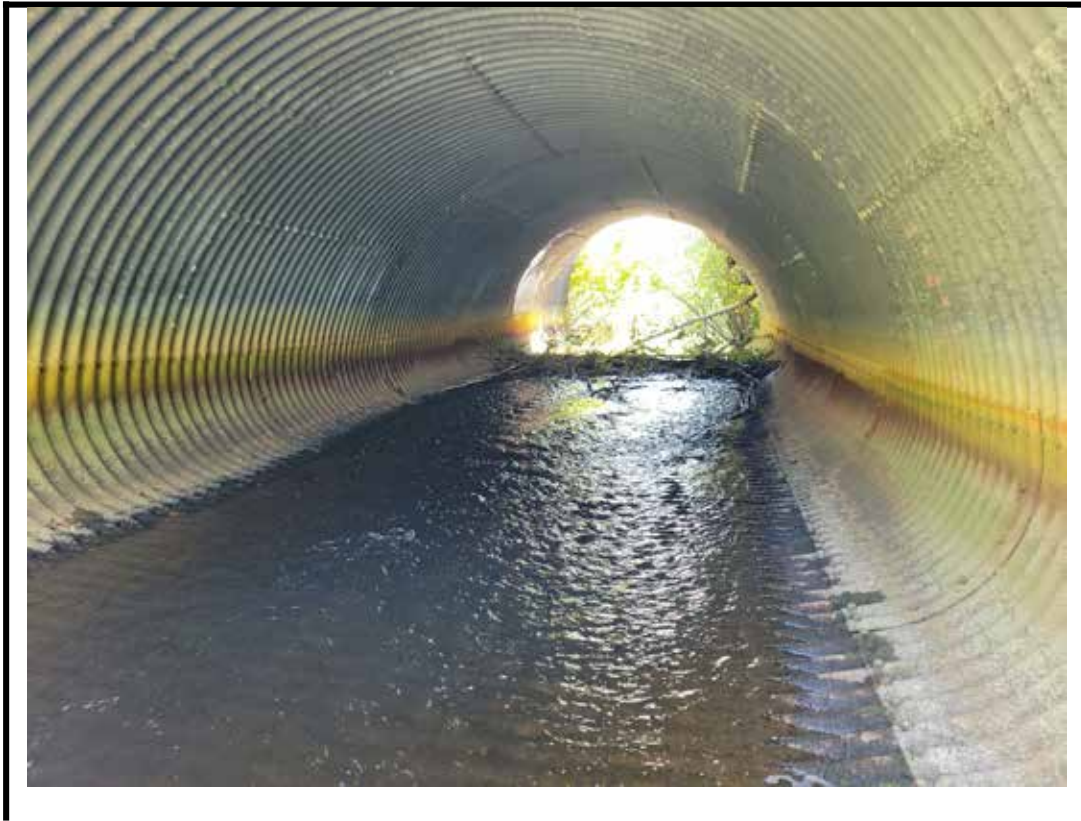
Photo 11 Interior of culvert barrel
