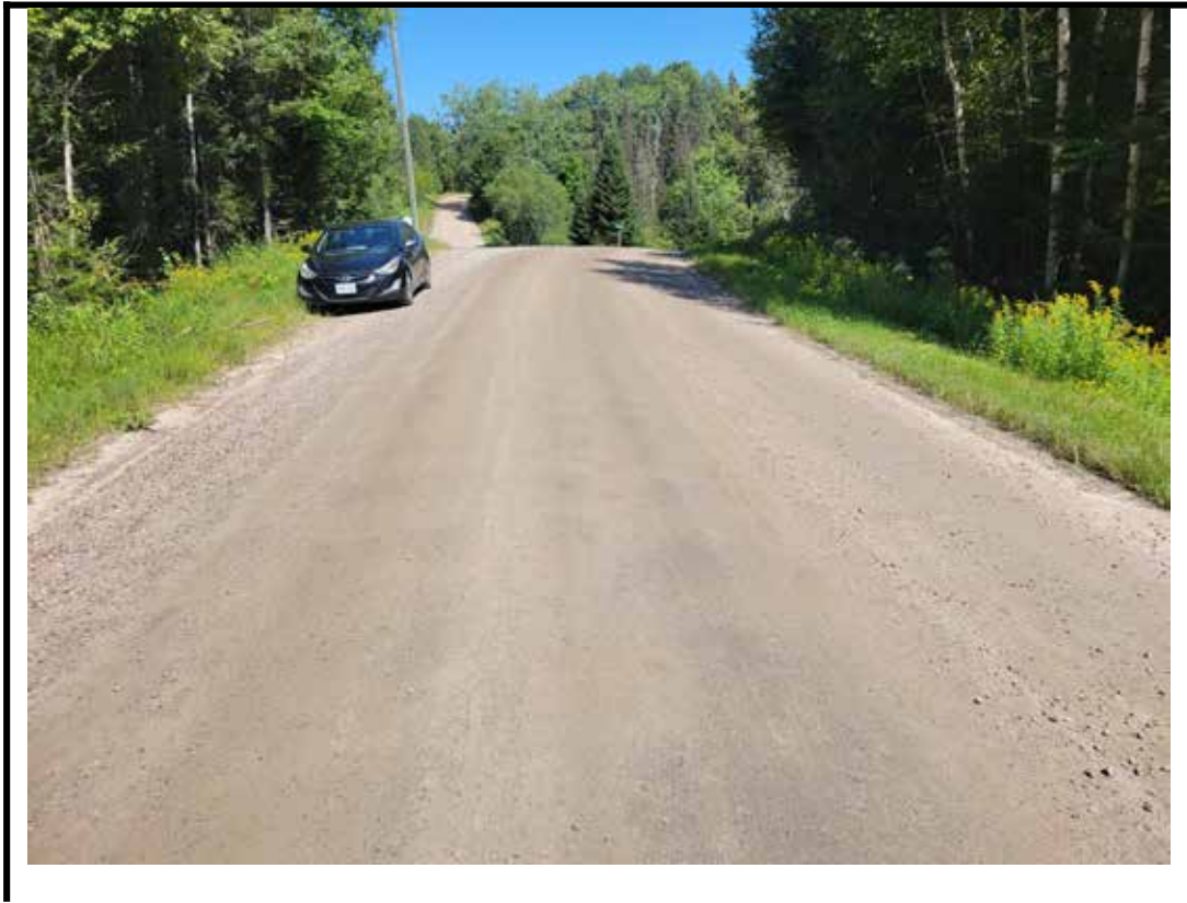
Photo 3 East approach from center of structure
