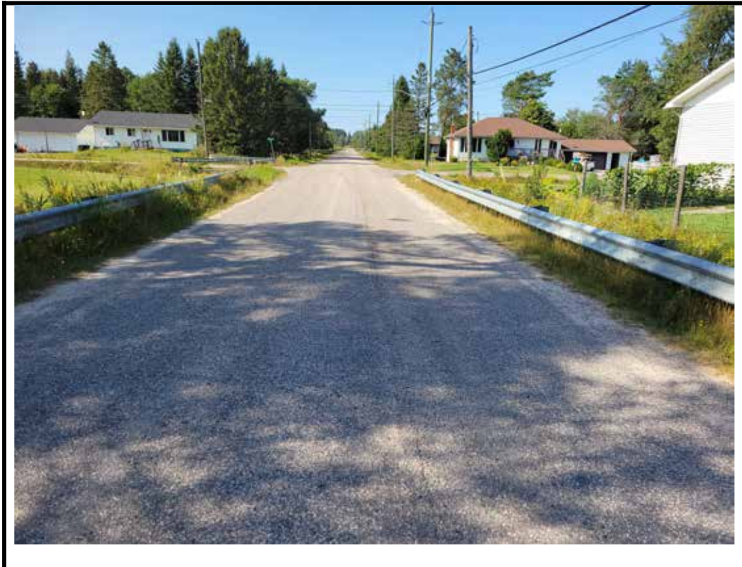
Photo 3 North approach from center of structure
