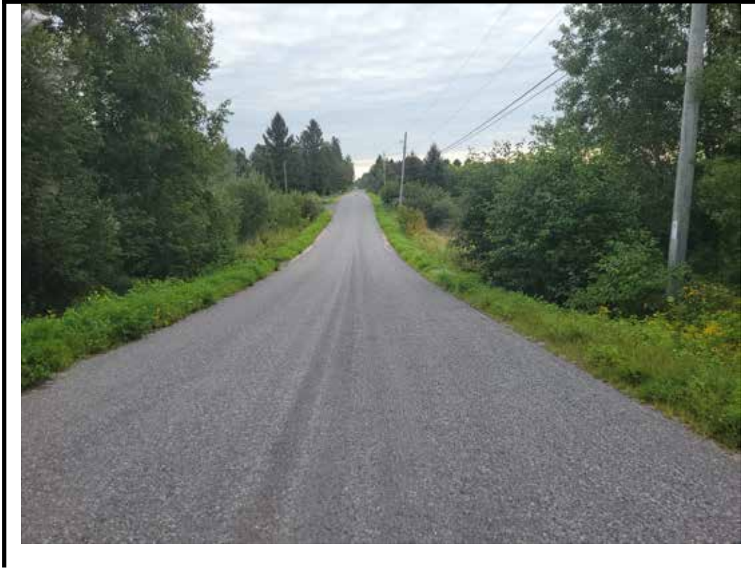
Photo 1 Structure from east approach
