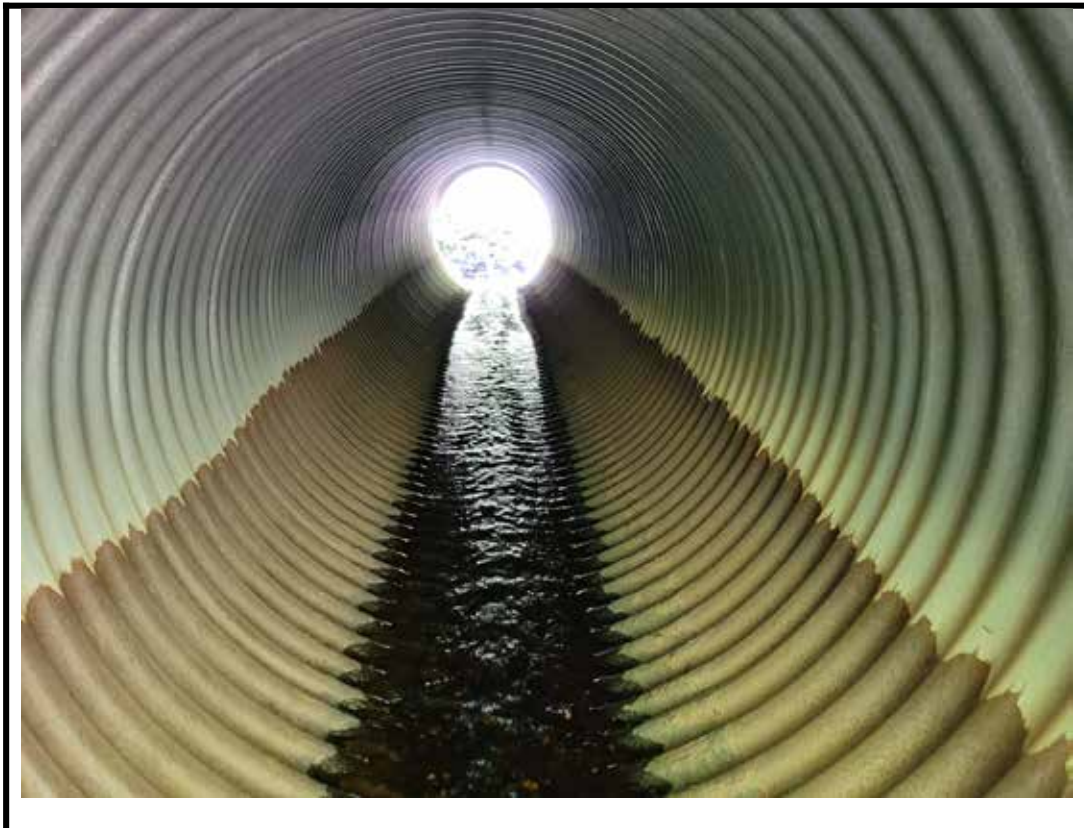
Photo 8 Interior of south barrel
