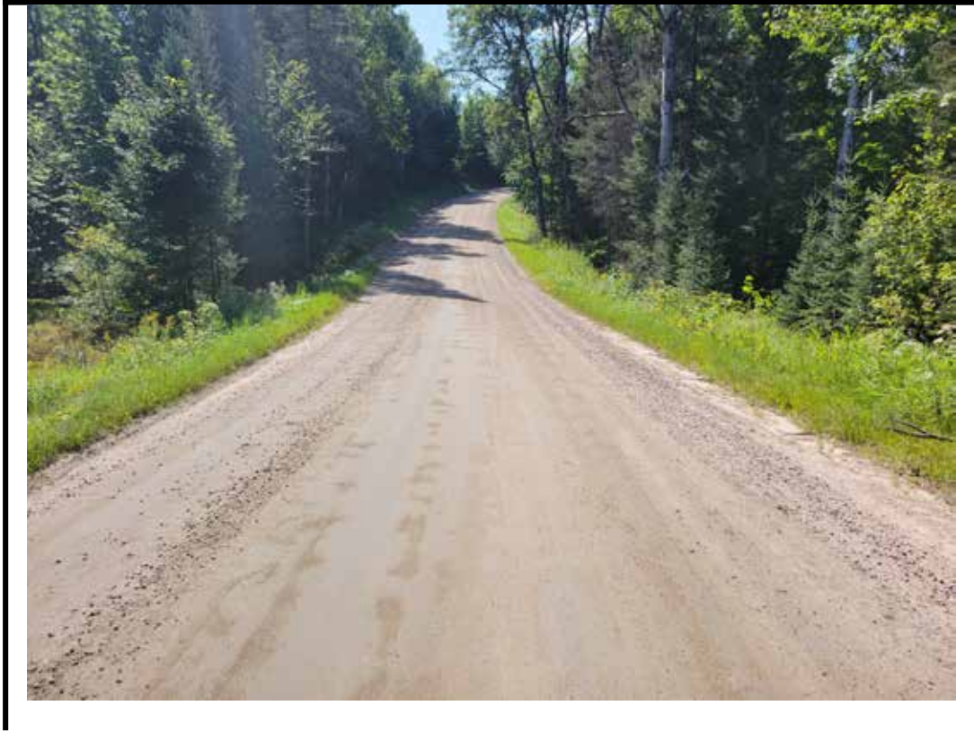
Photo 1 Structure from east approach
