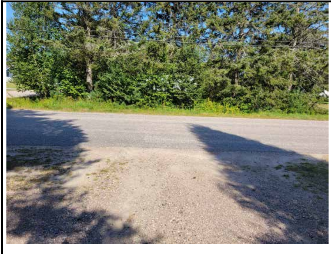
Photo 3 East approach from the center of structure
