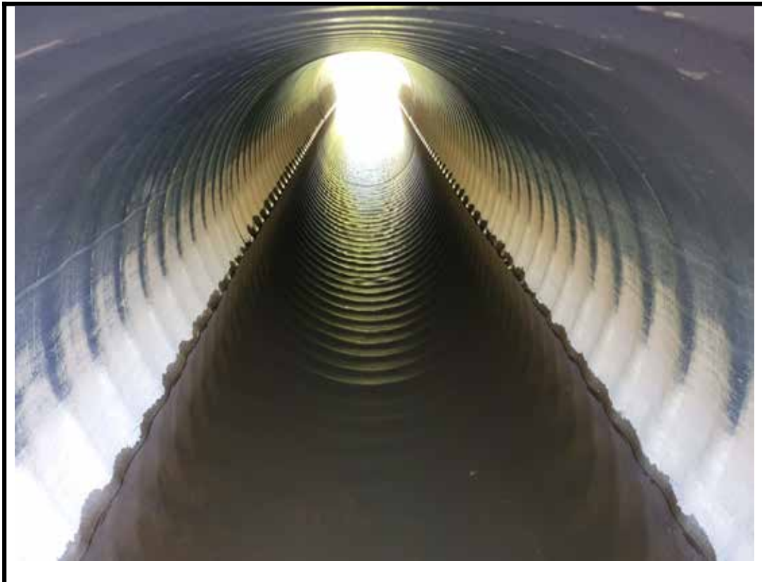
Photo 8 Interior of middle barrel; replaced since 2022 inspection
