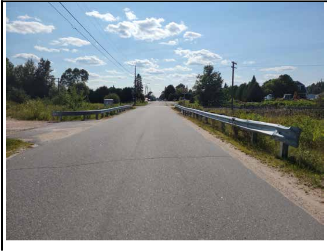
Photo 1 Structure from east approach
