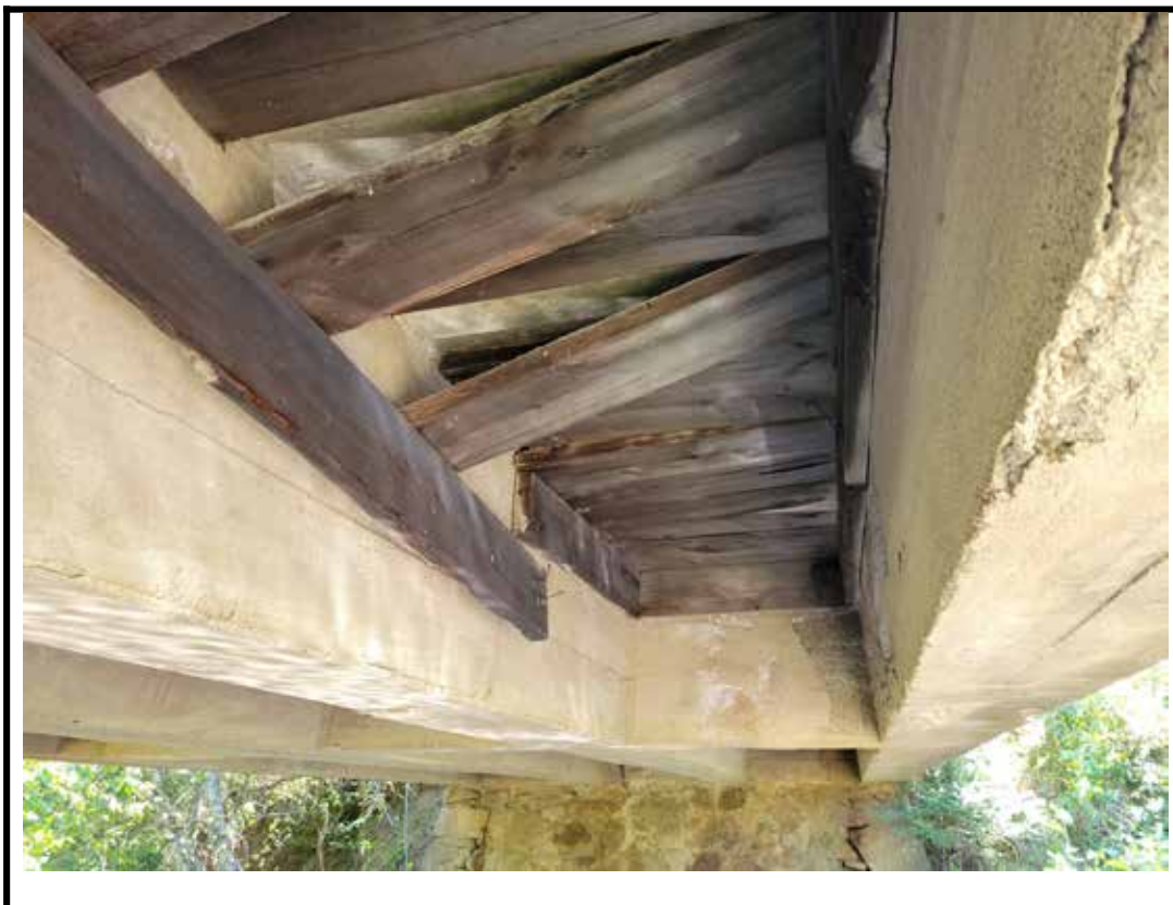
Photo 15 Timber formwork on north underside of deck
