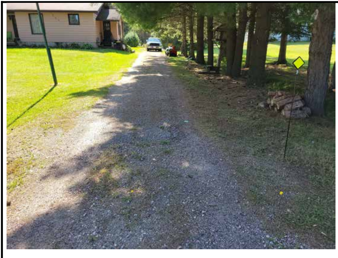
Photo 4 West approach from the center of structure
