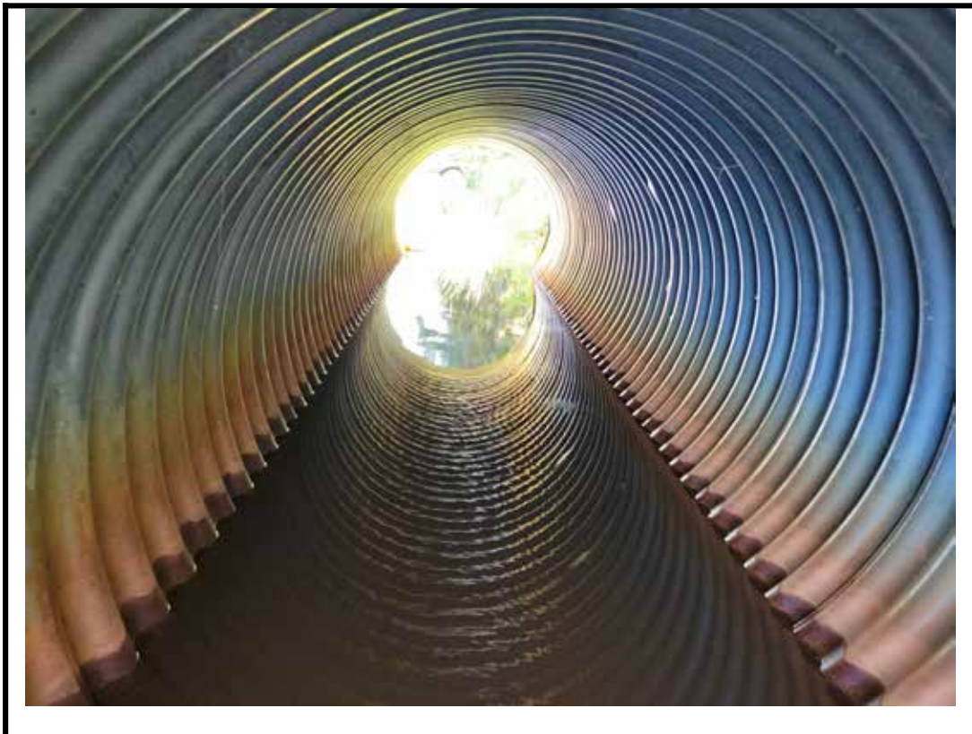
Photo 8 Interior of culvert barrel
