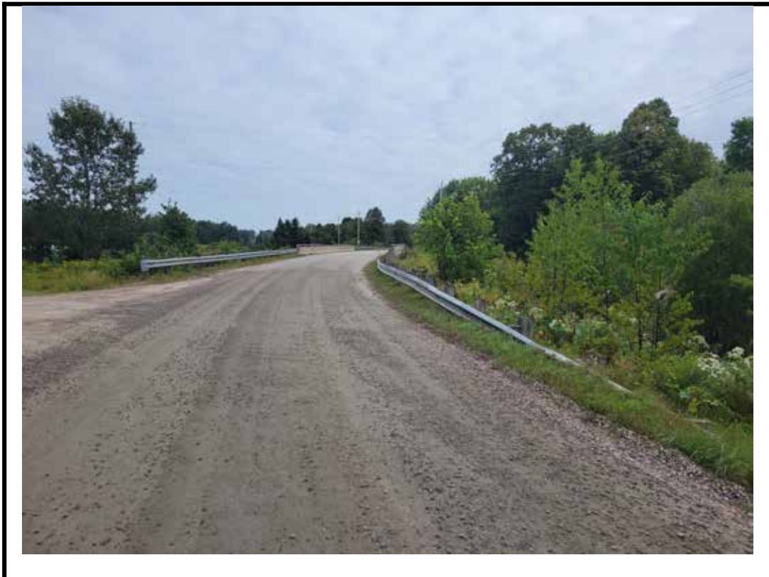
Photo 2 Structure from south approach
