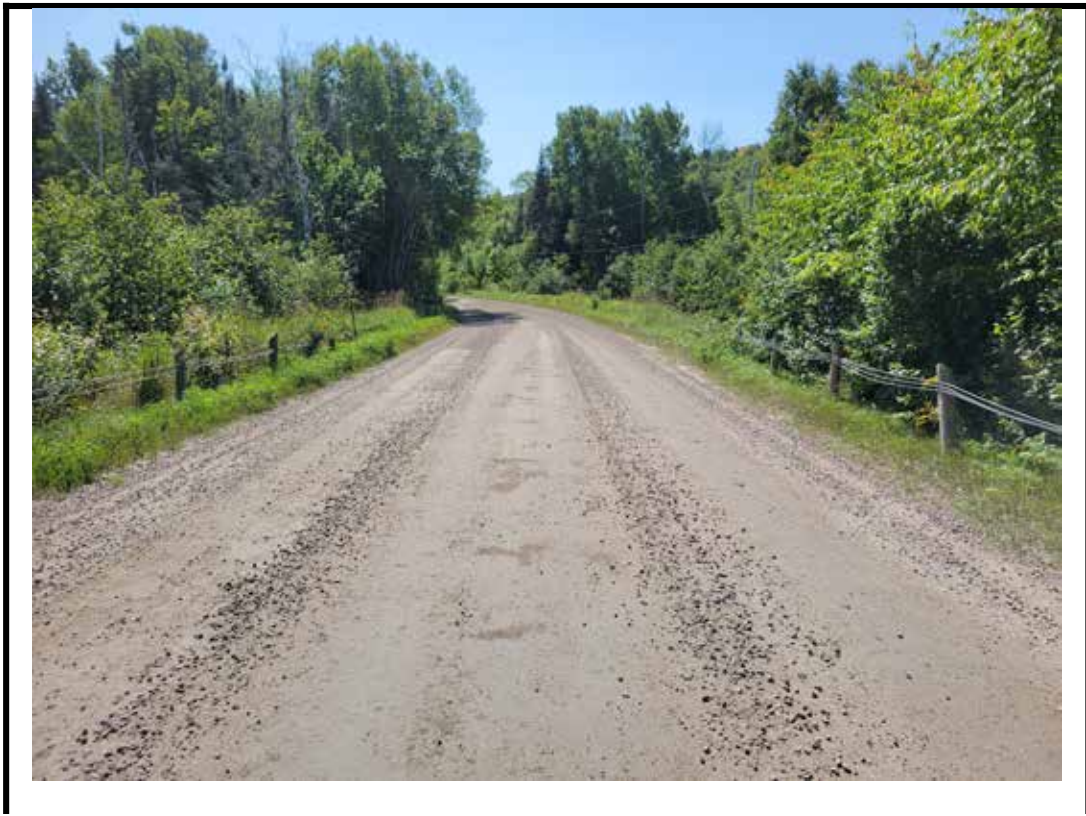
Photo 4 South approach from center of structure
