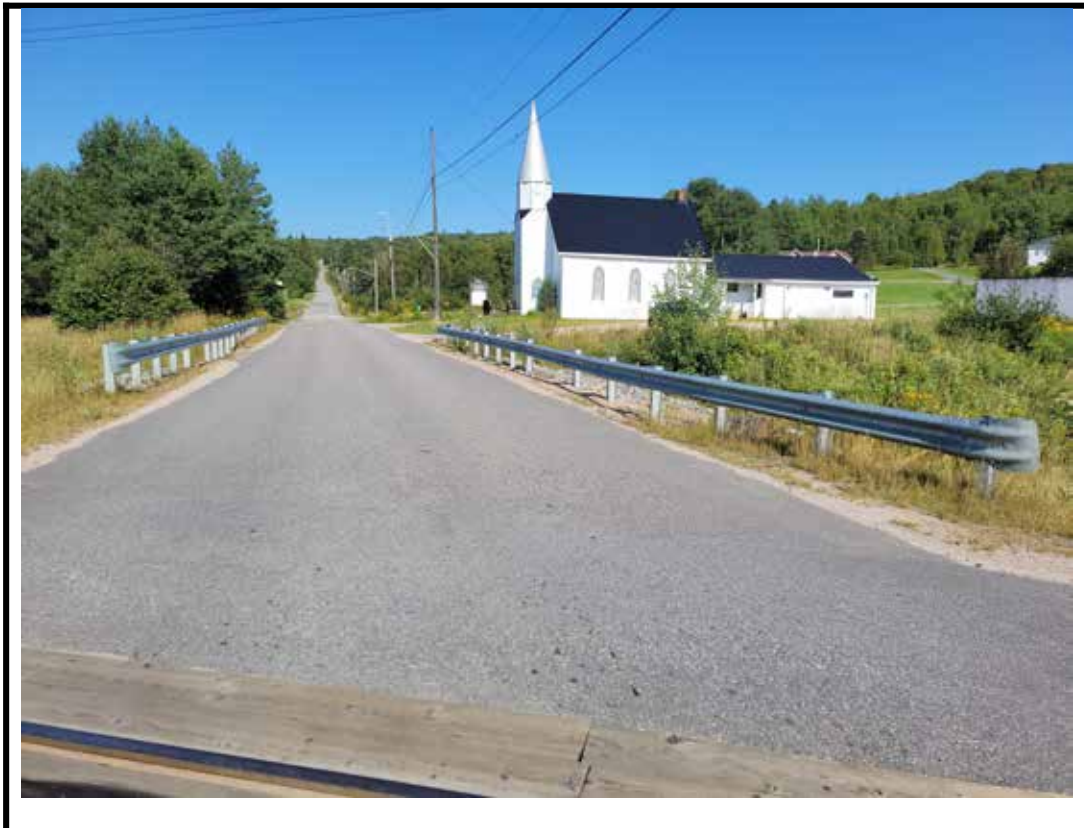
Photo 2 Structure from west approach
