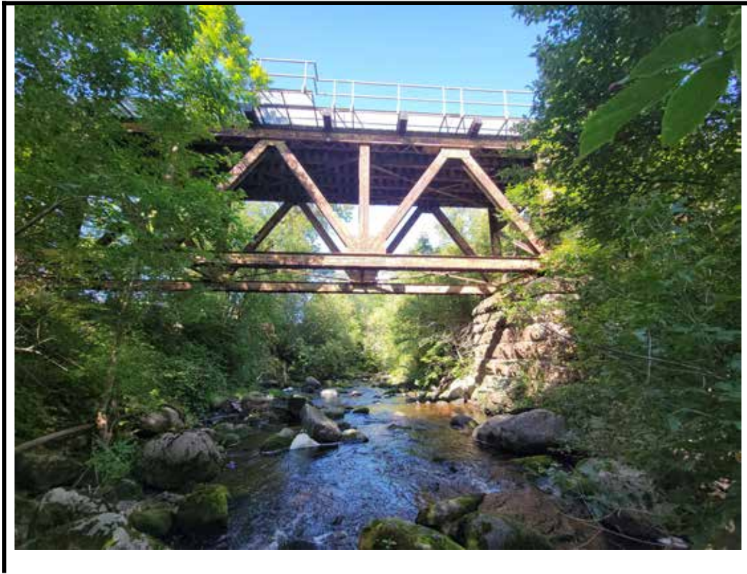
Photo 11 East elevation of center span
