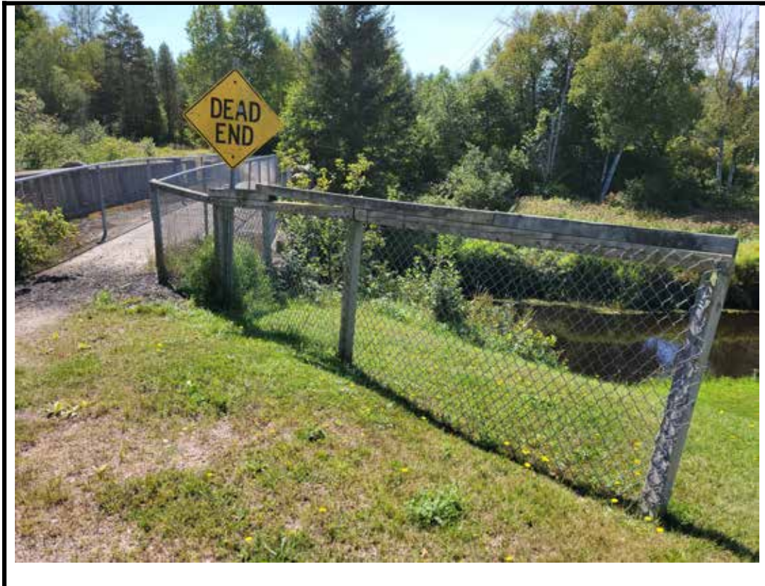
Photo 7 Dead end sign and chain link fence at east approach (Typical)
