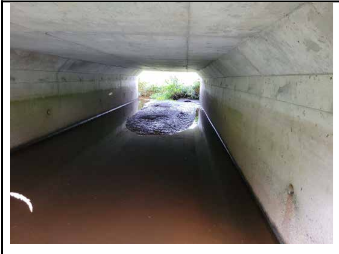
Photo 11 General view of barrel looking west
