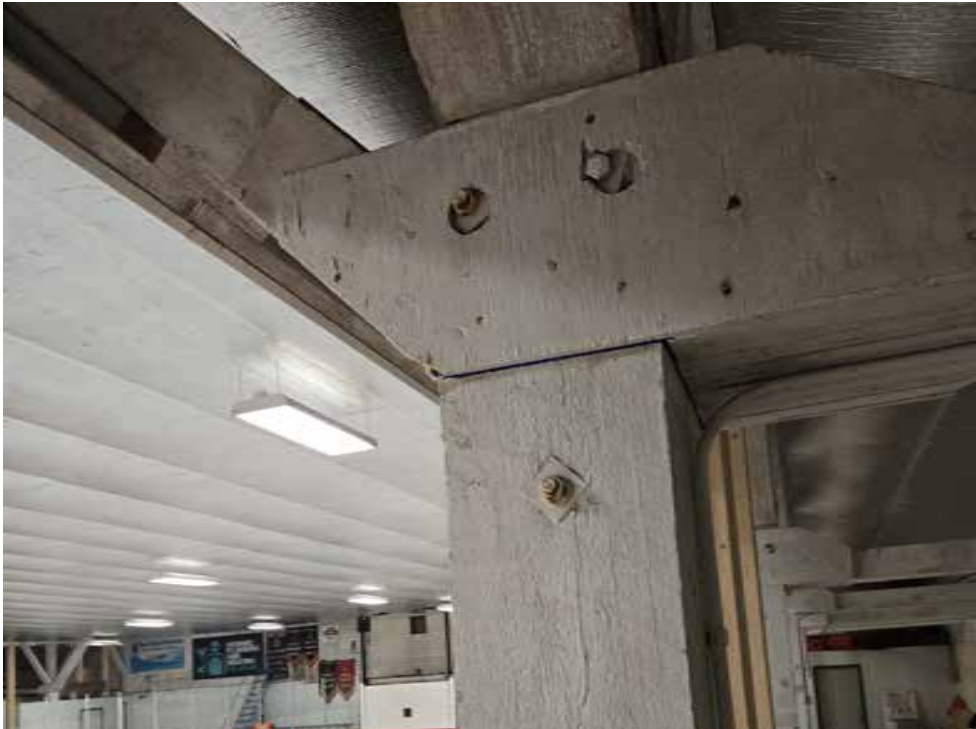
Photograph 10: Basic monitoring line at representative column location
