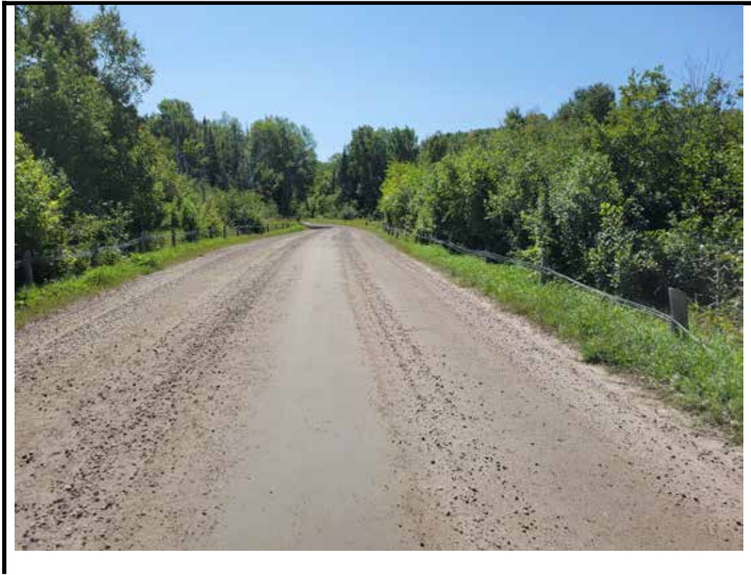
Photo 1 Structure from north approach
