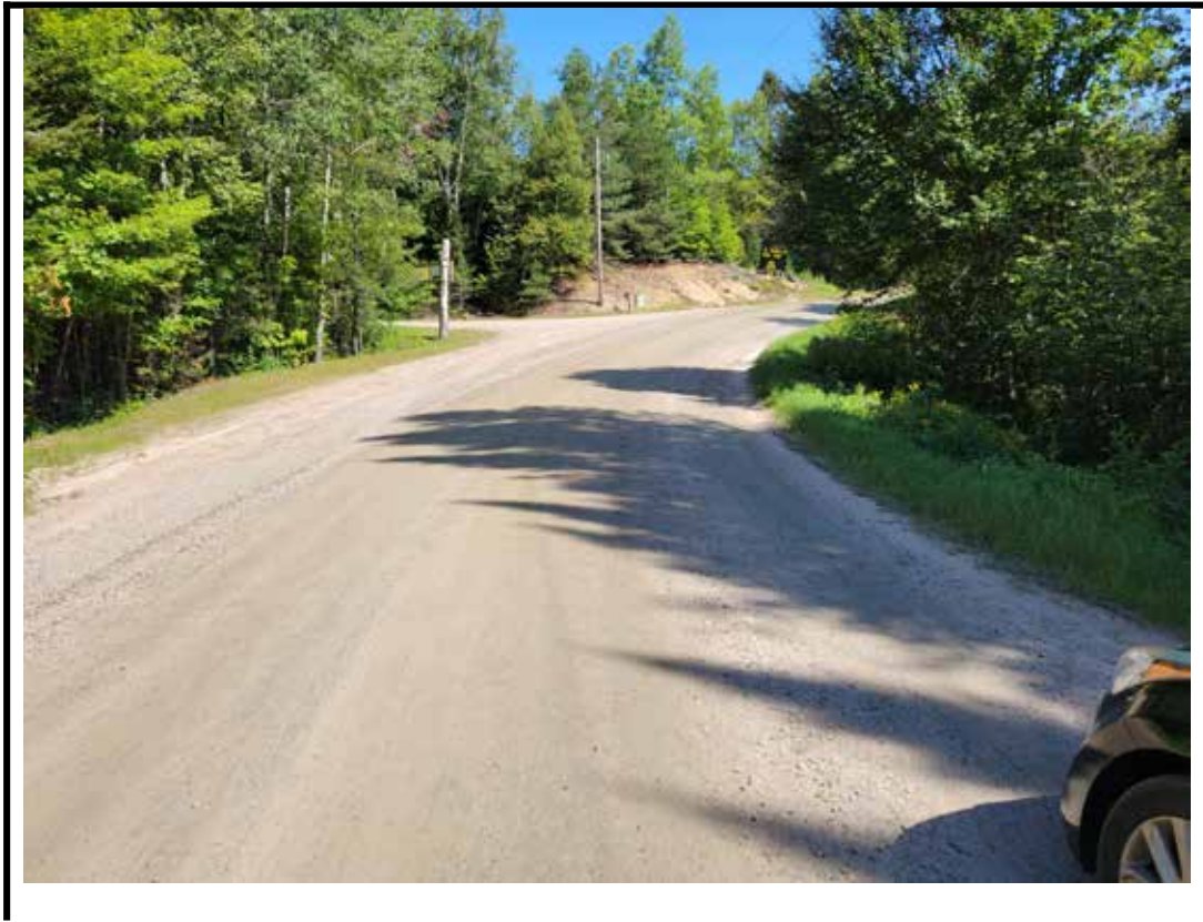
Photo 1 Structure from north approach
