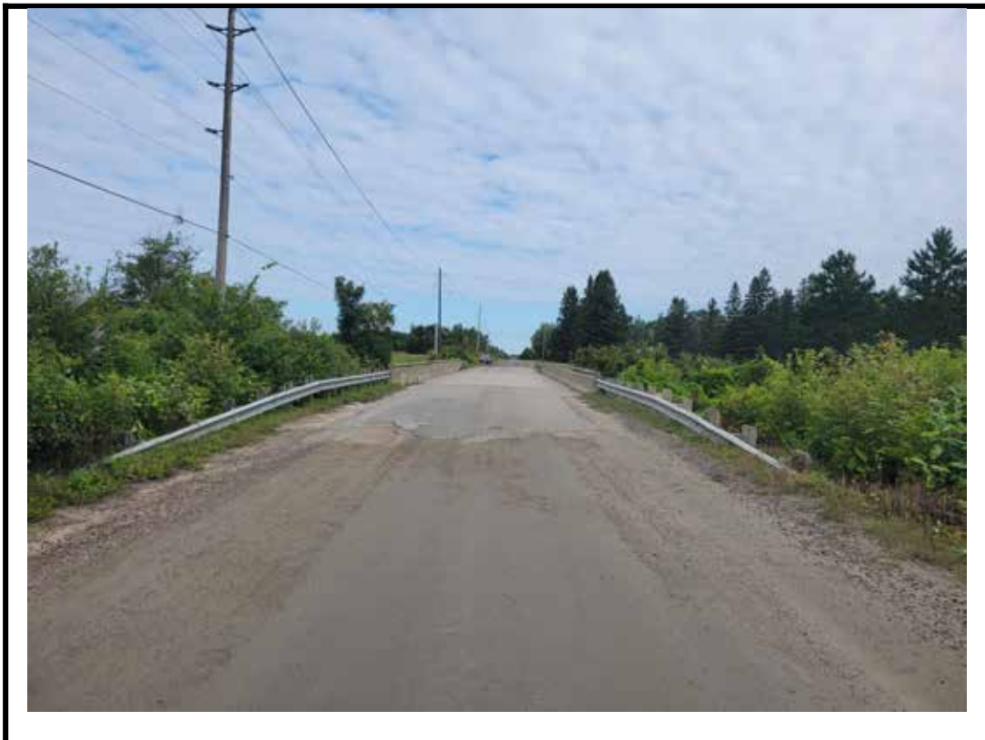
Photo 2 Structure from south approach
