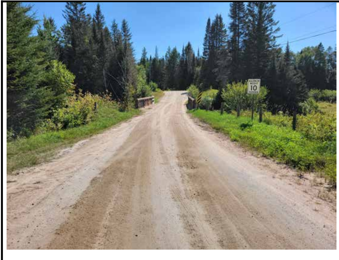
Photo 1 Structure from north approach
