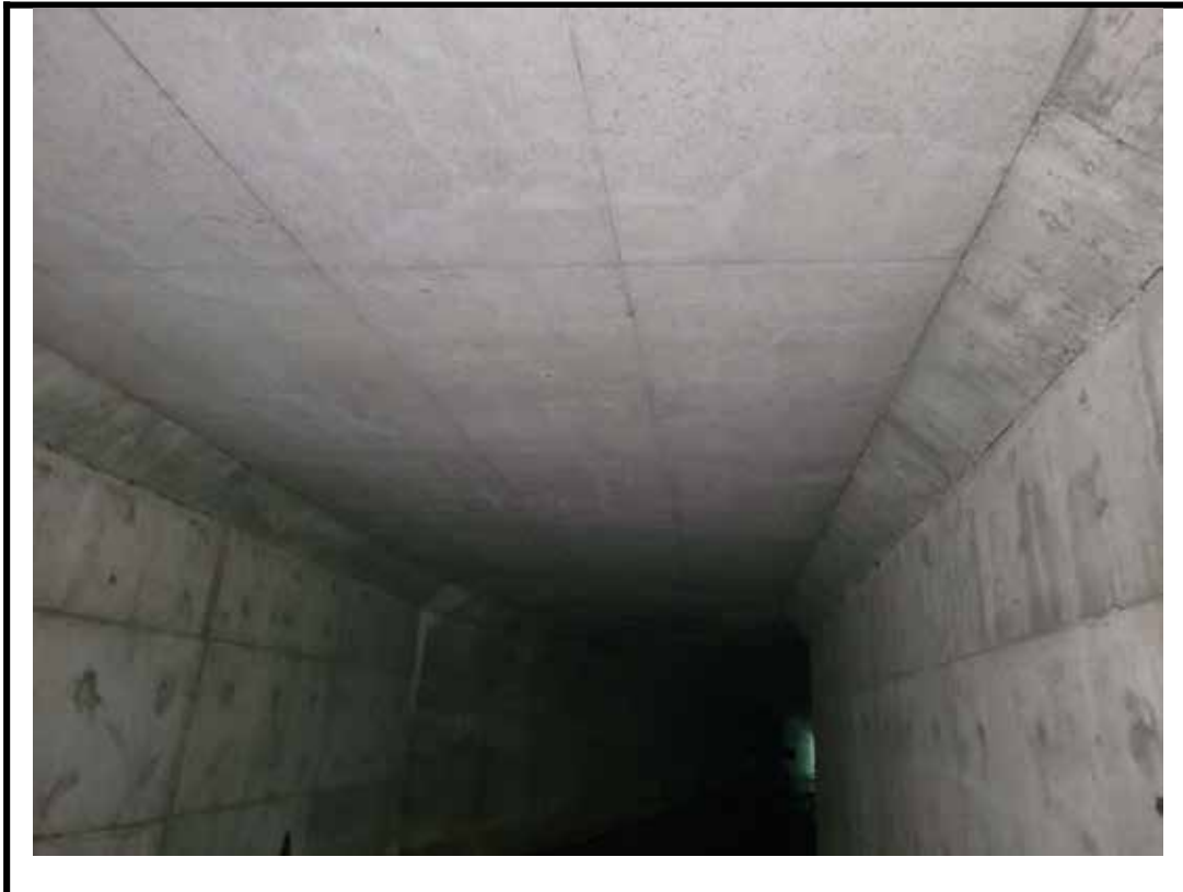
Photo 9 General view of east end of barrel
