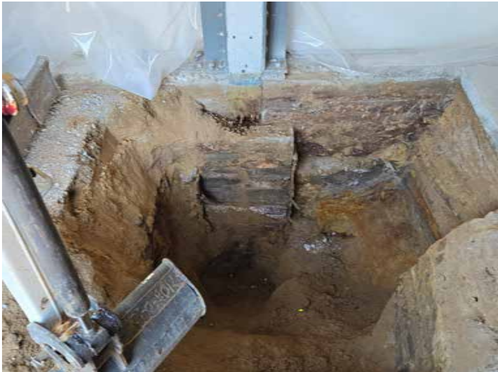
Photograph 2: Concrete pier adjacent foundation wall - interior
