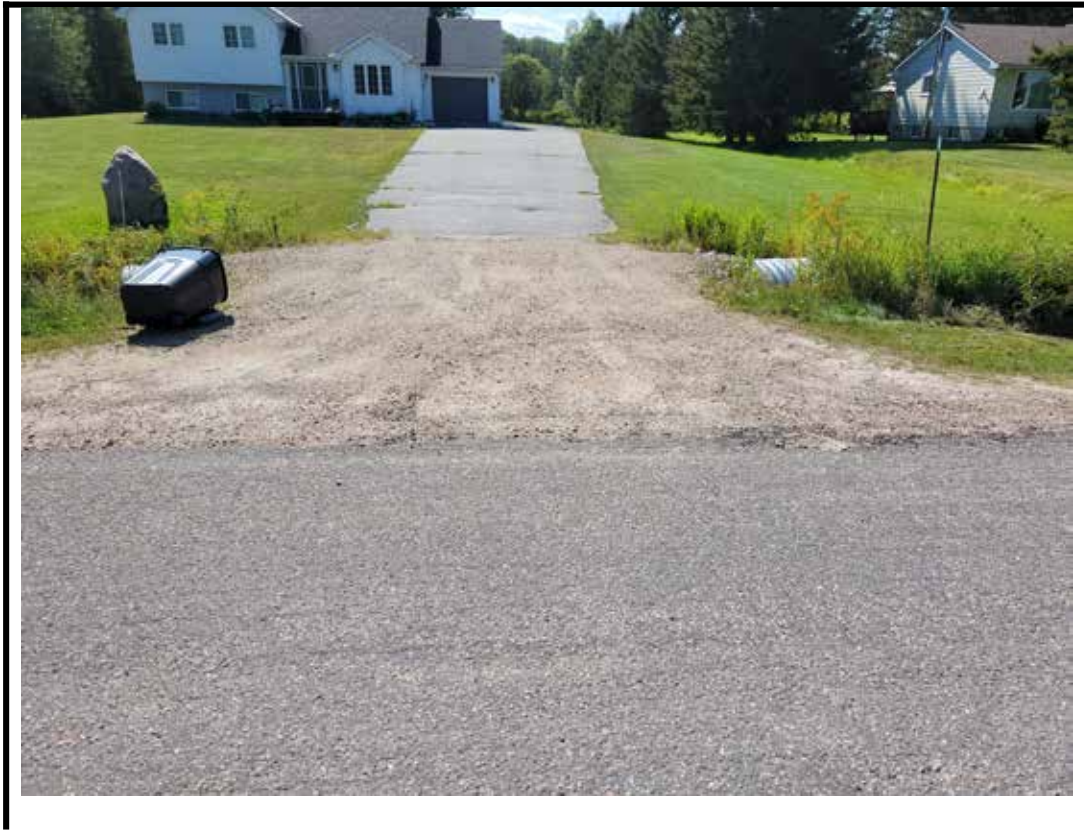
Photo 1 Structure from East approach
