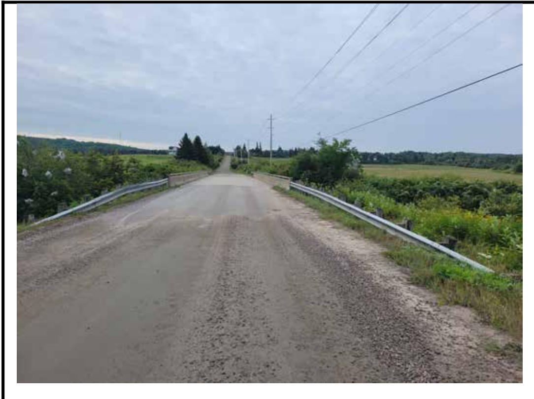
Photo 1 Structure from north approach
