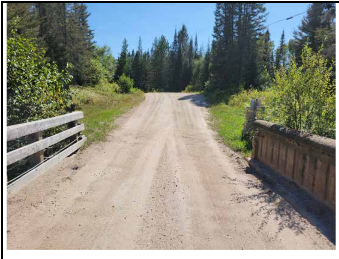
Photo 4 South approach from center of structure
