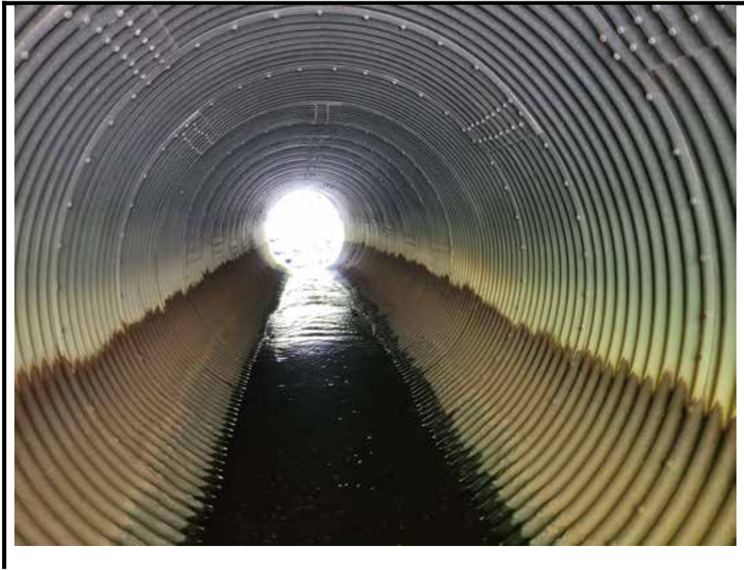
Photo 7 Interior of north barrel
