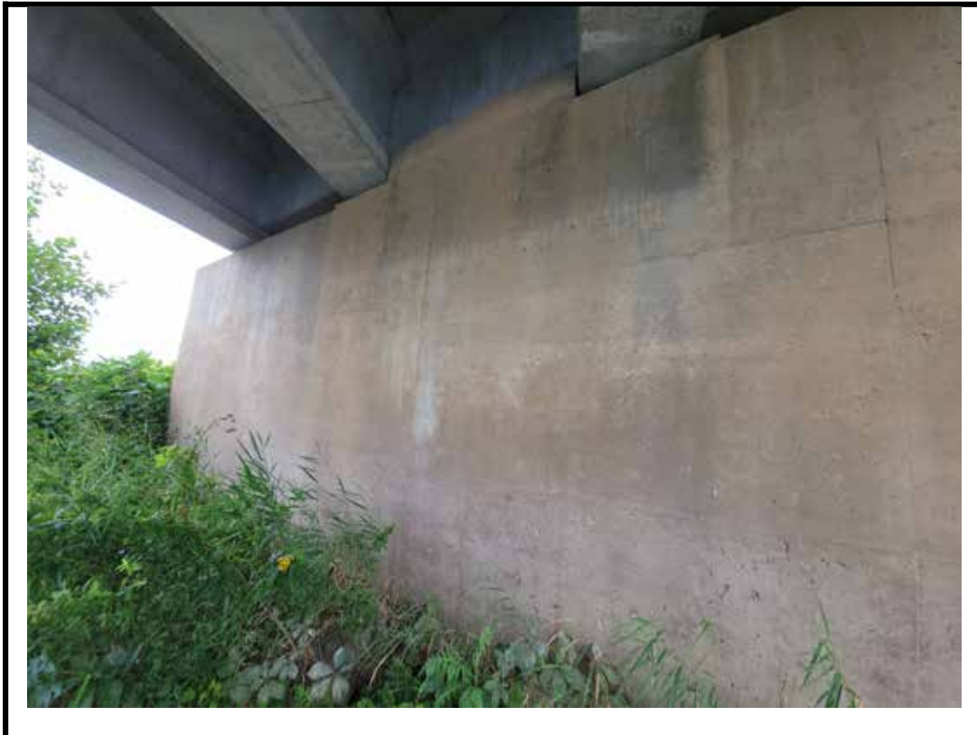
Photo 14 General view of abutment wall
