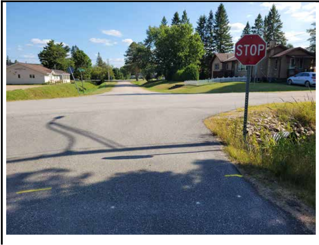
Photo 1 Structure from north approach
