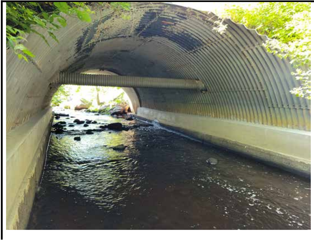
Photo 11 Concrete repair on bottom section of barrel
