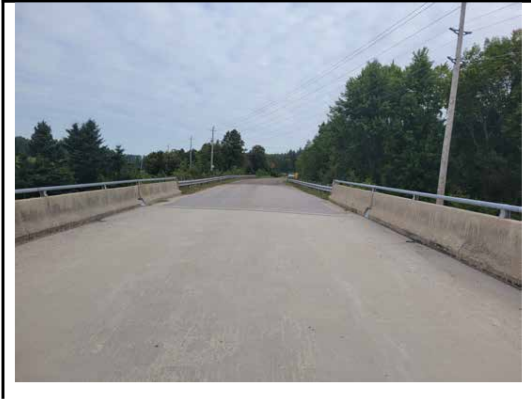
Photo 3 North approach from center of structure
