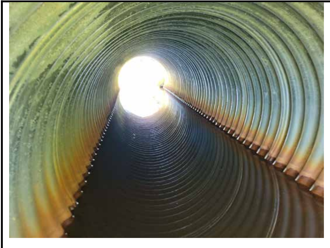
Photo 7 Typical view of interior barrel
