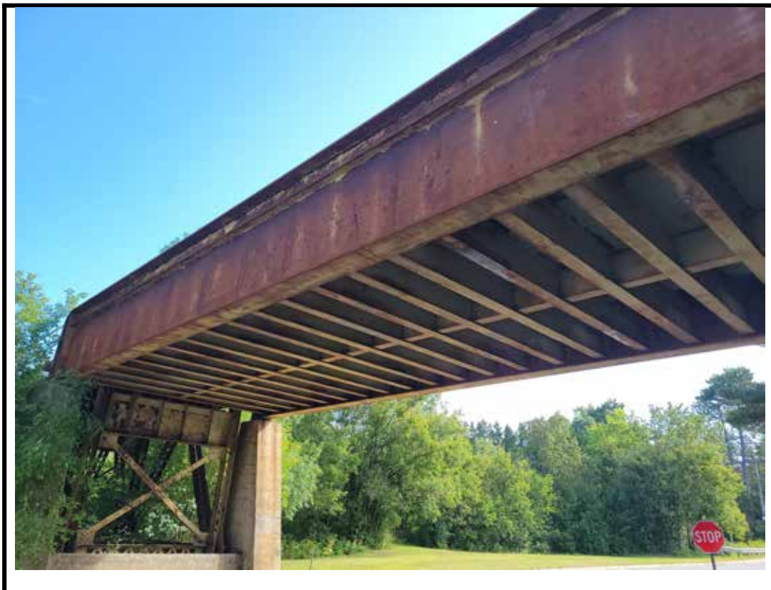
Photo 8 South underside of structure
