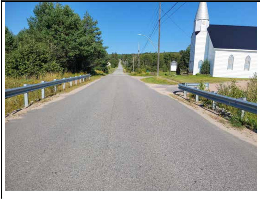
Photo 3 East approach from center of structure
