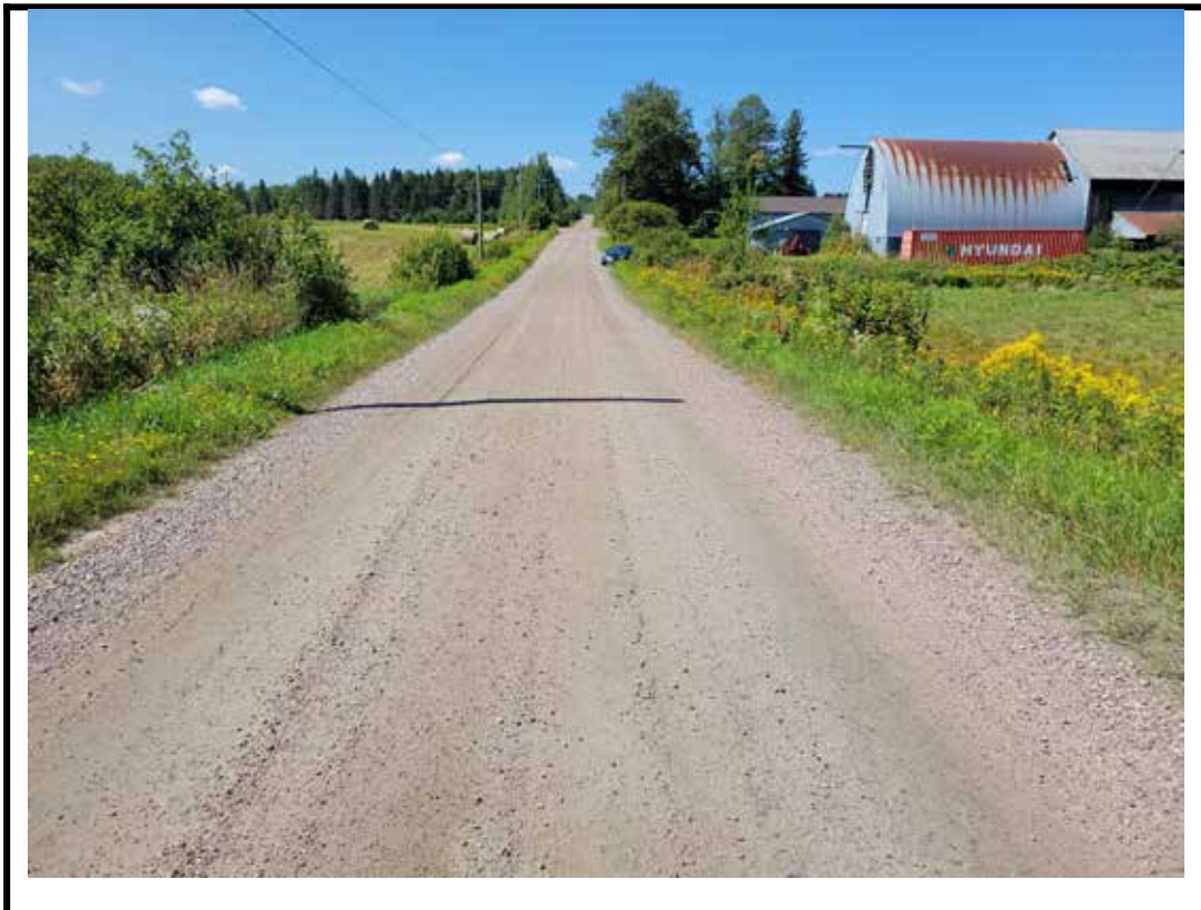
Photo 4 West approach from center of structure
