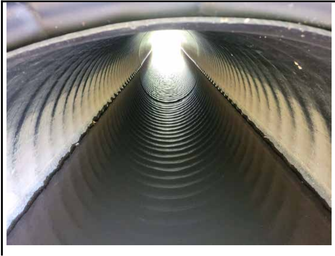
Photo 9 Interior of west barrel; replaced since 2022 inspection
