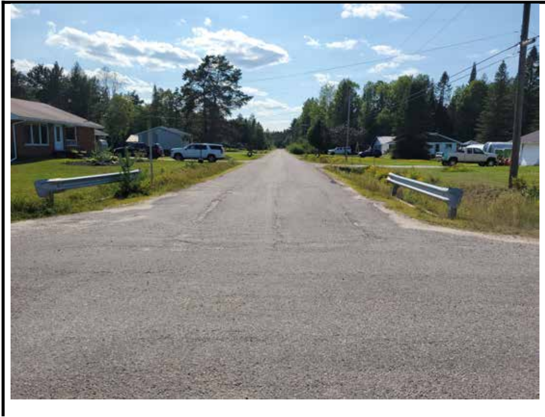
Photo 1 Structure from east approach
