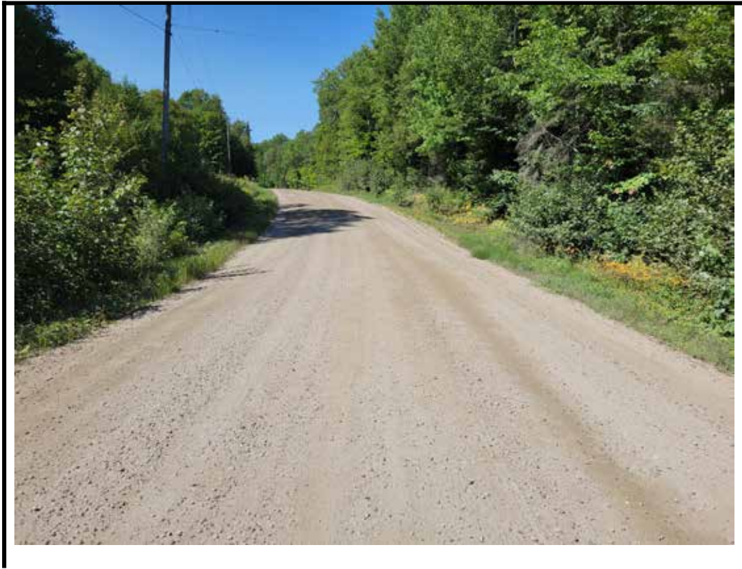
Photo 3 North approach from center of structure
