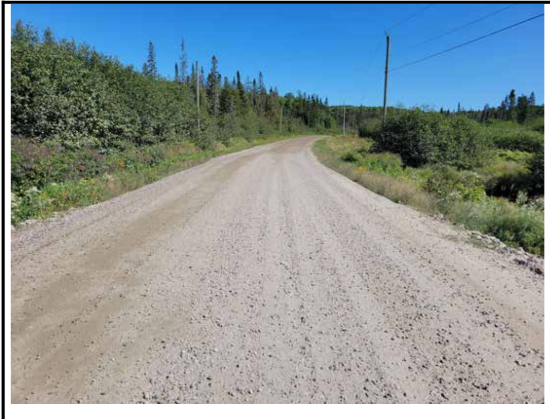
Photo 4 West approach from center of structure
