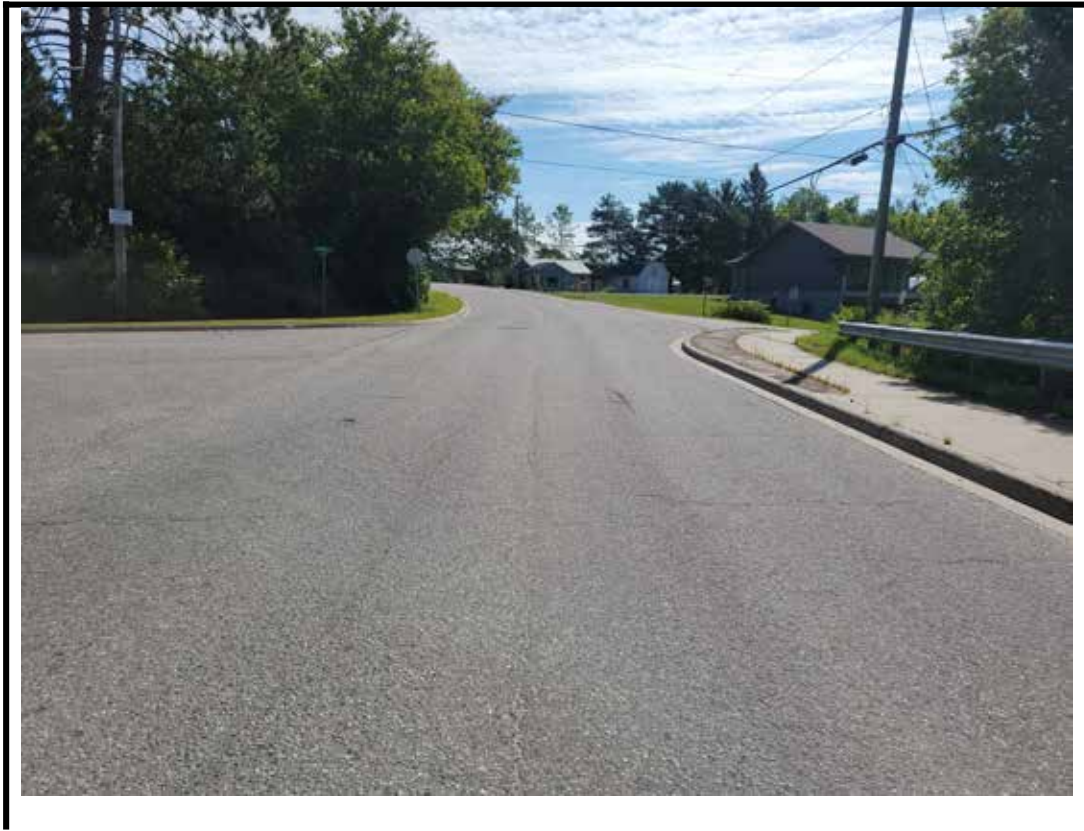
Photo 3 East approach from center of structure
