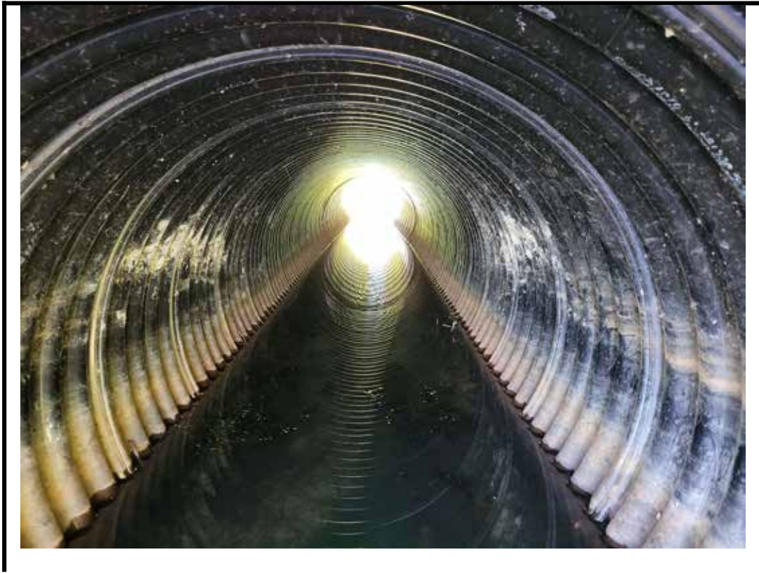
Photo 7 Interior of culvert barrel looking south
