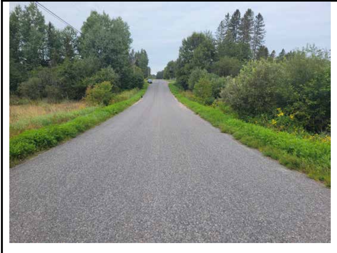
Photo 2 Structure from west approach
