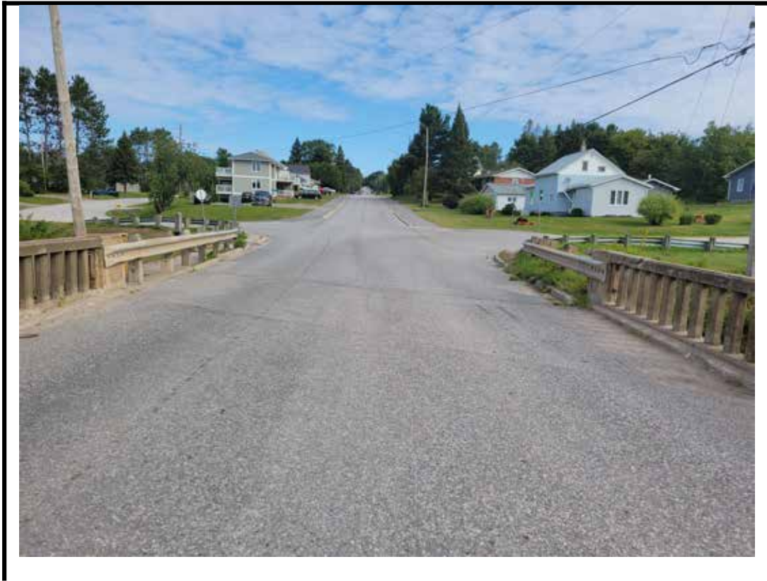
Photo 3 North approach from center of structure
