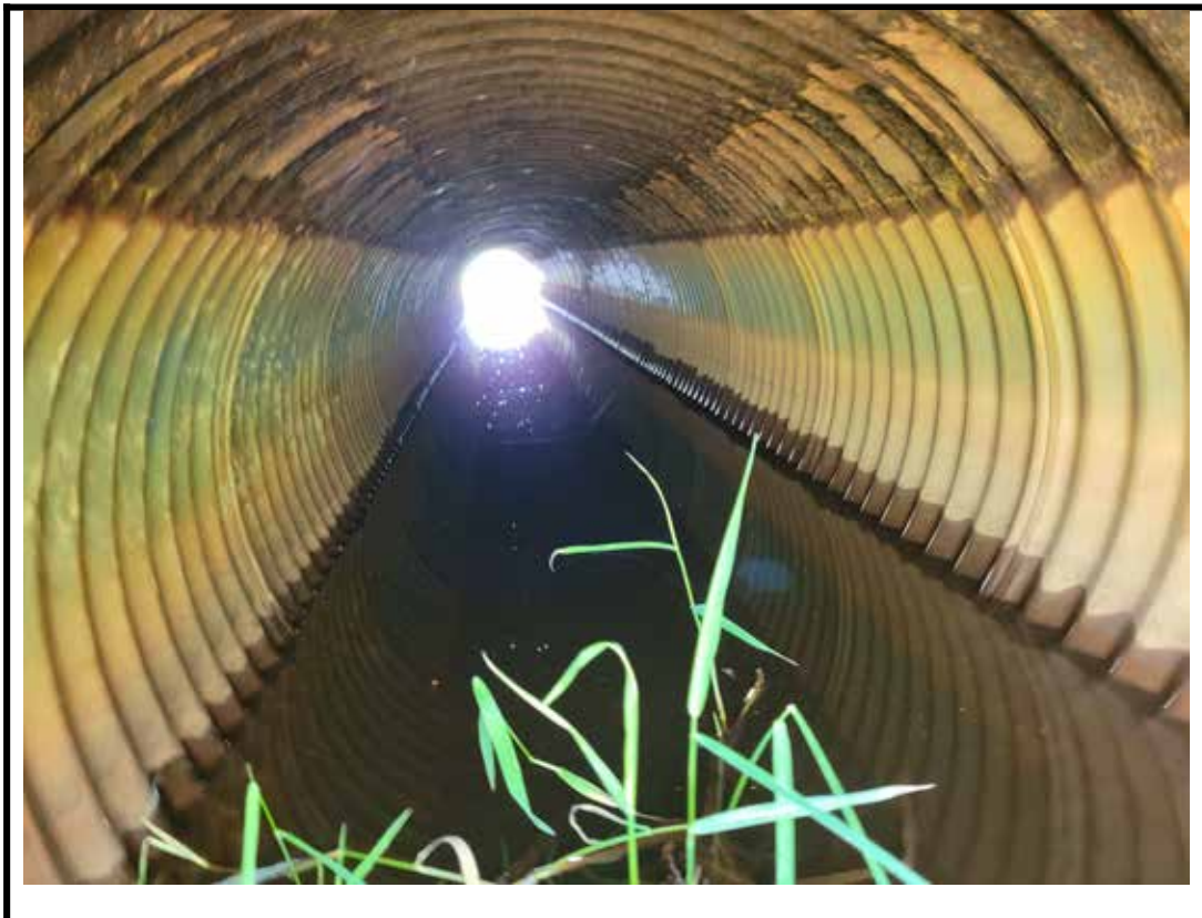
Photo 8 Interior of west culvert barrel
