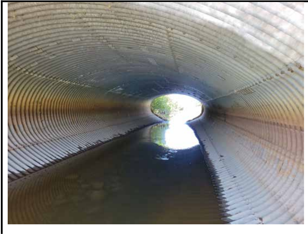
Photo 7 General condition of barrel looking north
