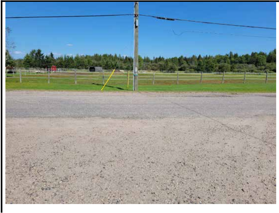
Photo 3 East approach from the center of structure
