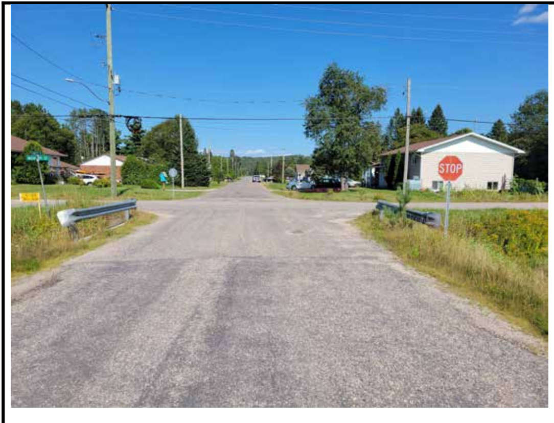
Photo 2 Structure from west approach
