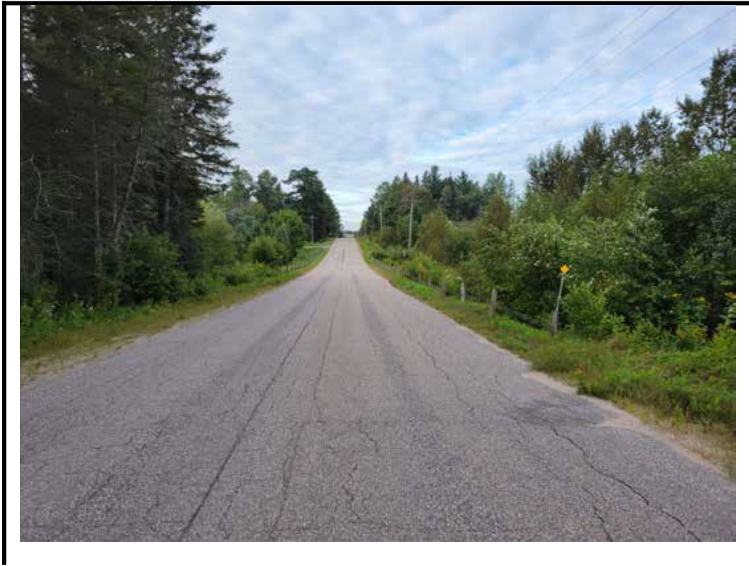
Photo 1 Structure from north approach
