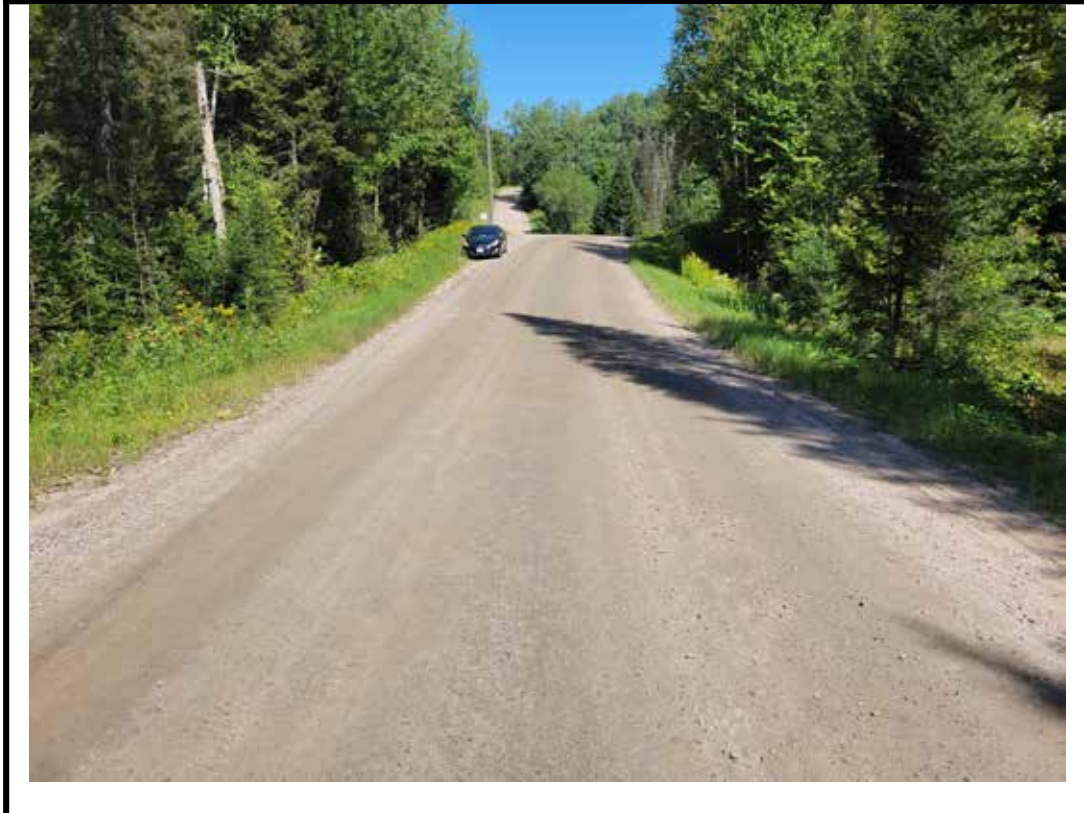
Photo 2 Structure from west approach
