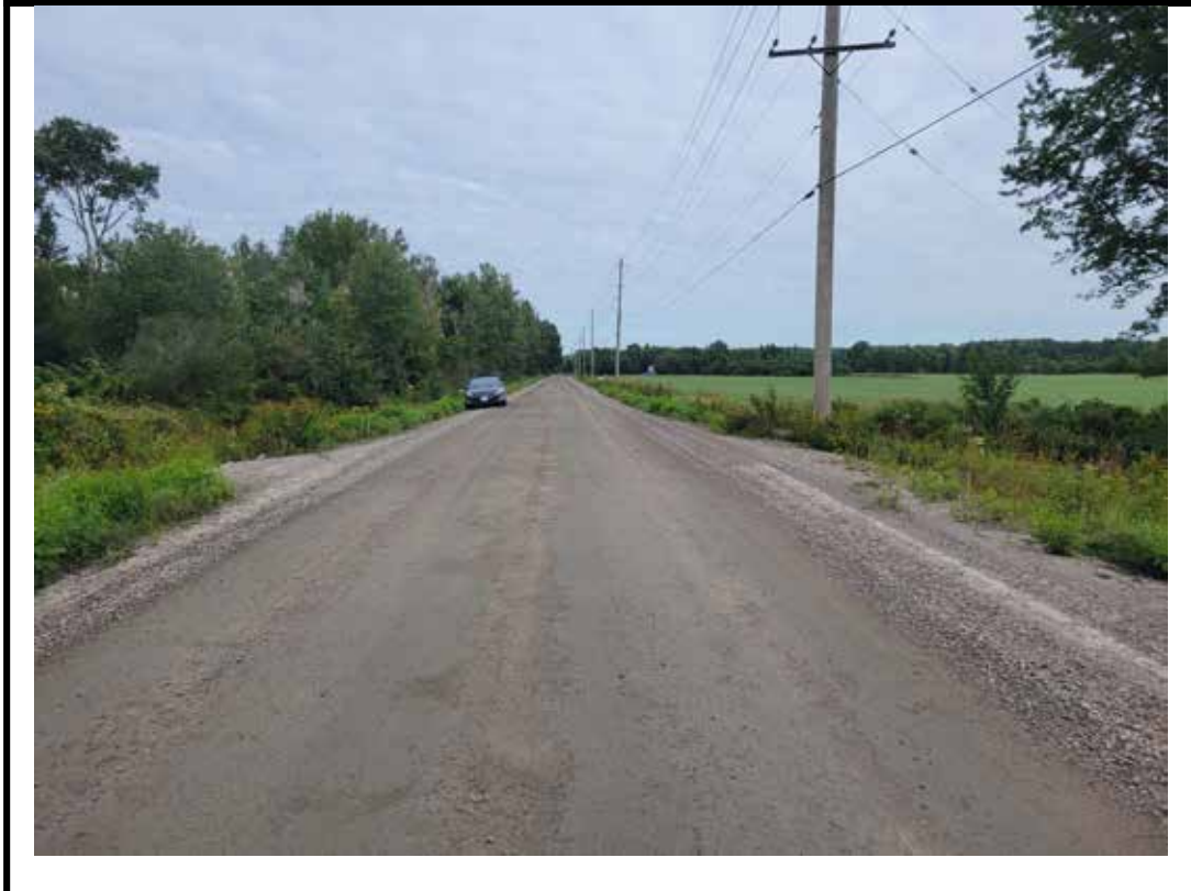
Photo 2 Structure from south approach
