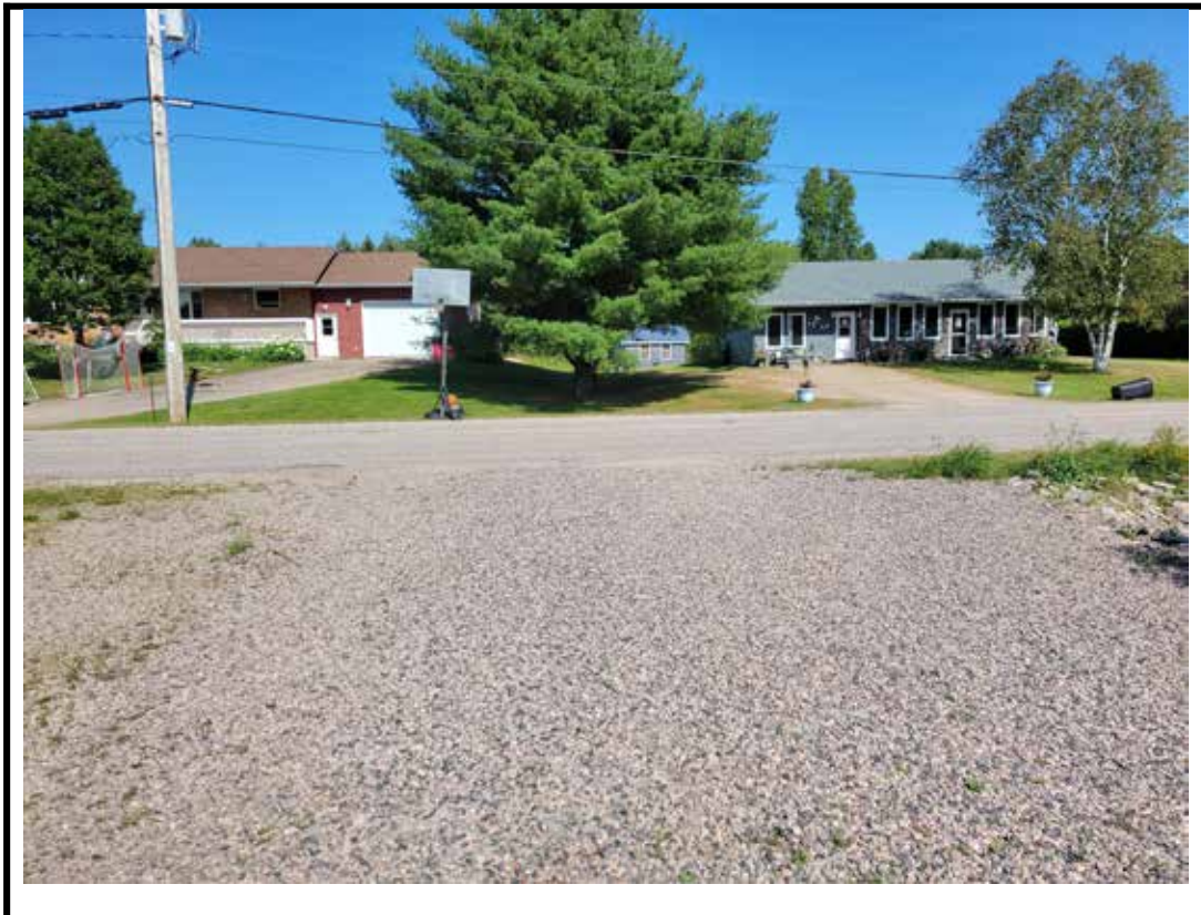
Photo 2 Structure from West approach
