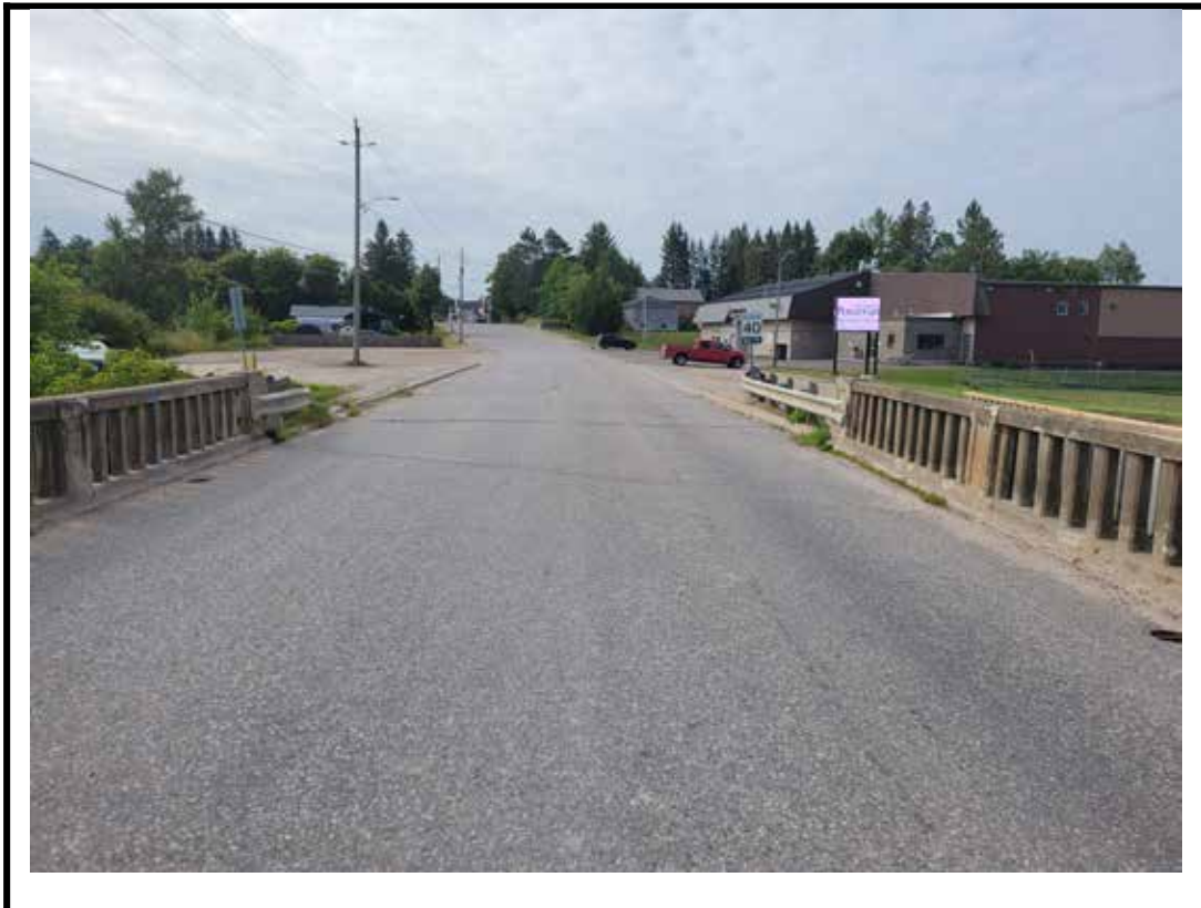
Photo 4 South approach from center of structure
