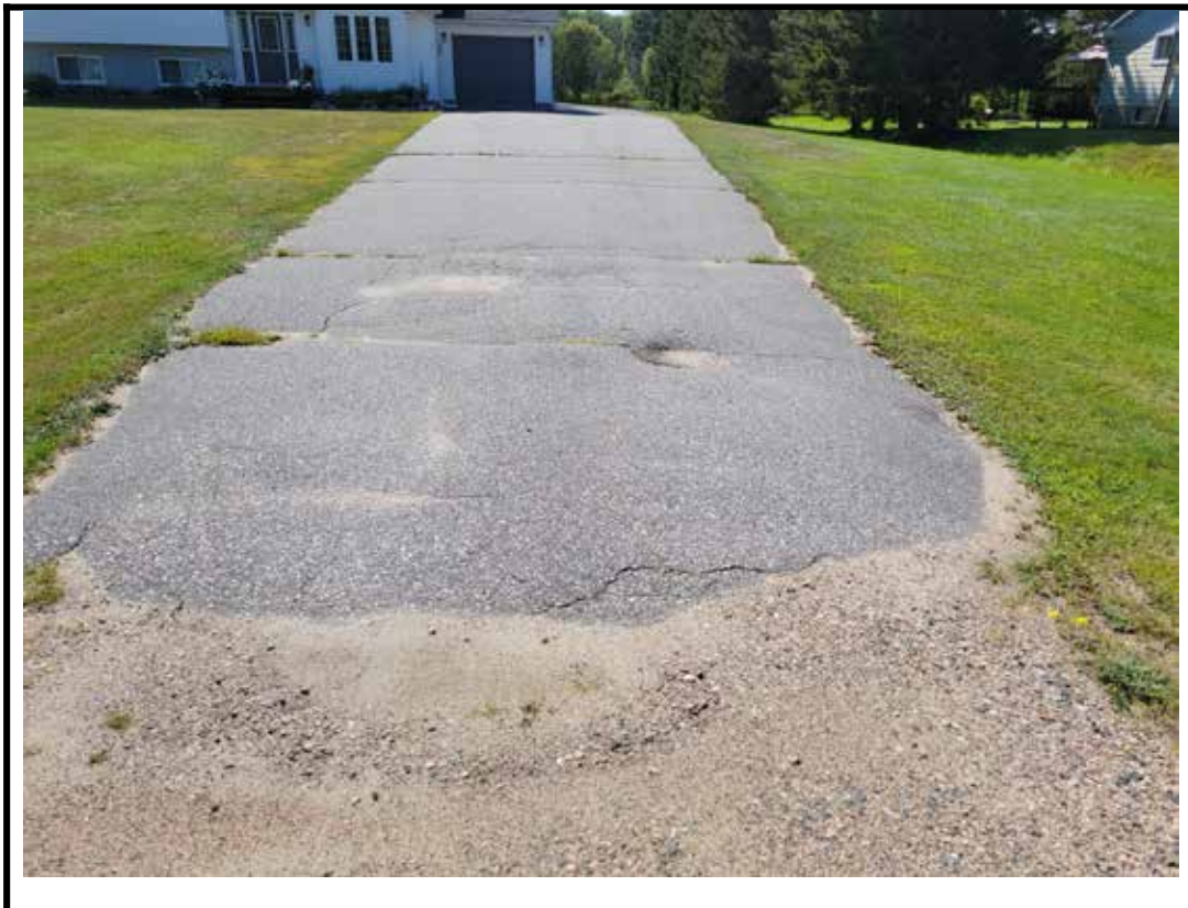
Photo 4 West approach from the center of structure
