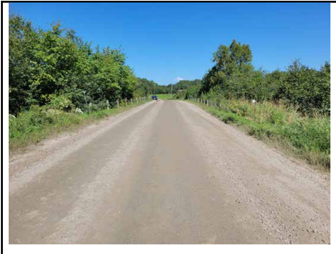
Photo 2 Structure from south approach
