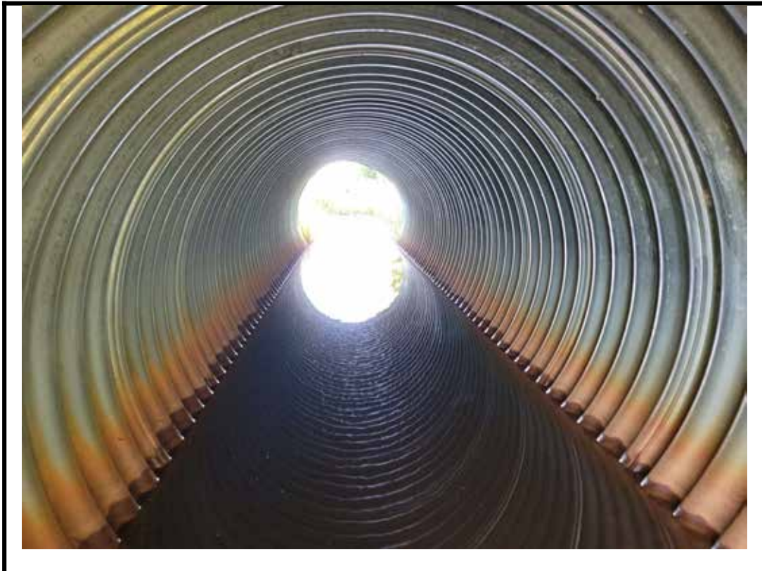
Photo 8 Typical view of culvert barrel
