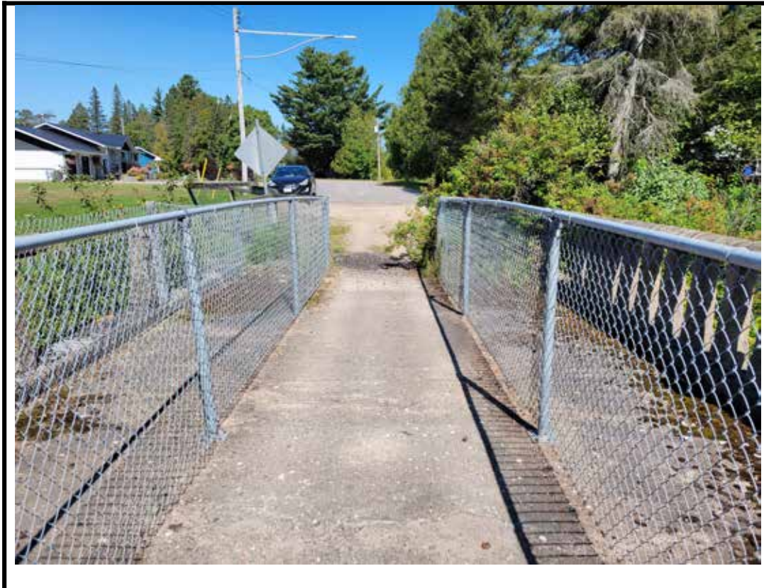
Photo 3 East approach from center of structure
