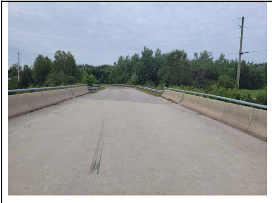
Photo 4 South approach from center of structure
