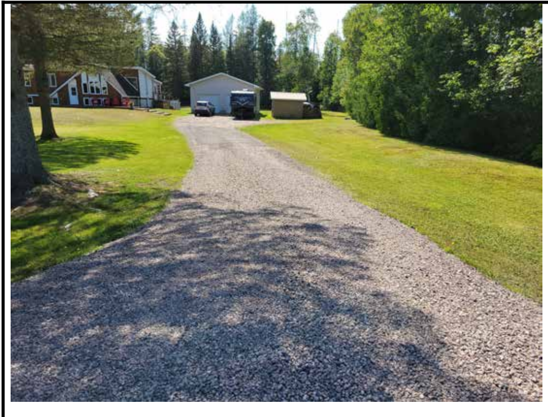
Photo 4 West approach from the center of structure
