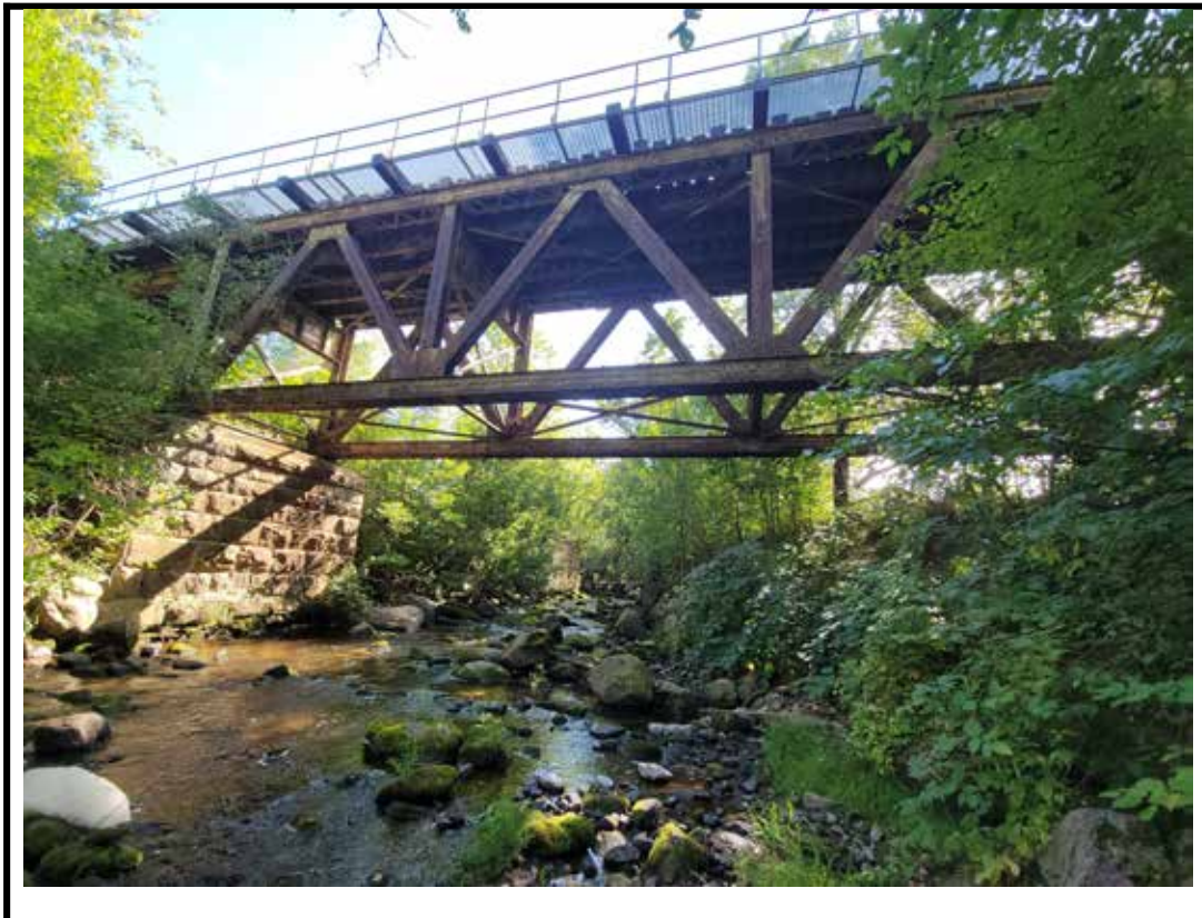
Photo 12 West elevation of center span
