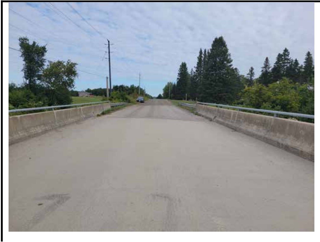
Photo 3 North approach from center of structure
