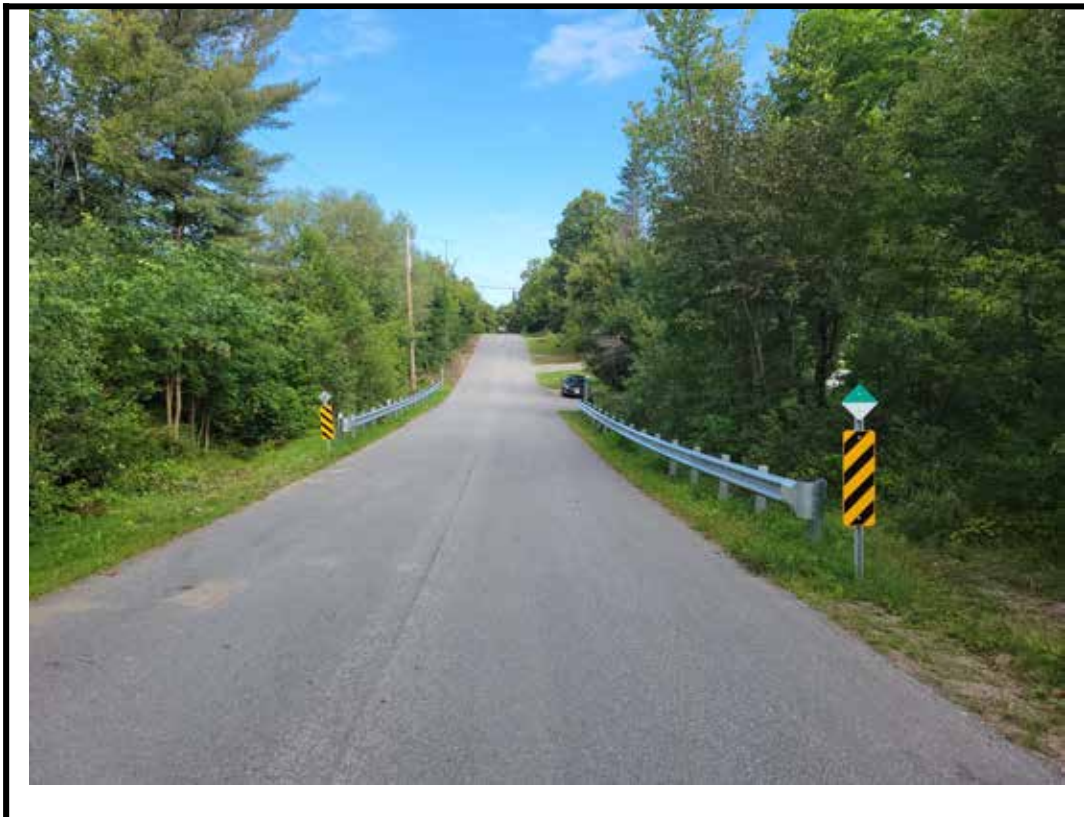
Photo 2 Structure from south approach
