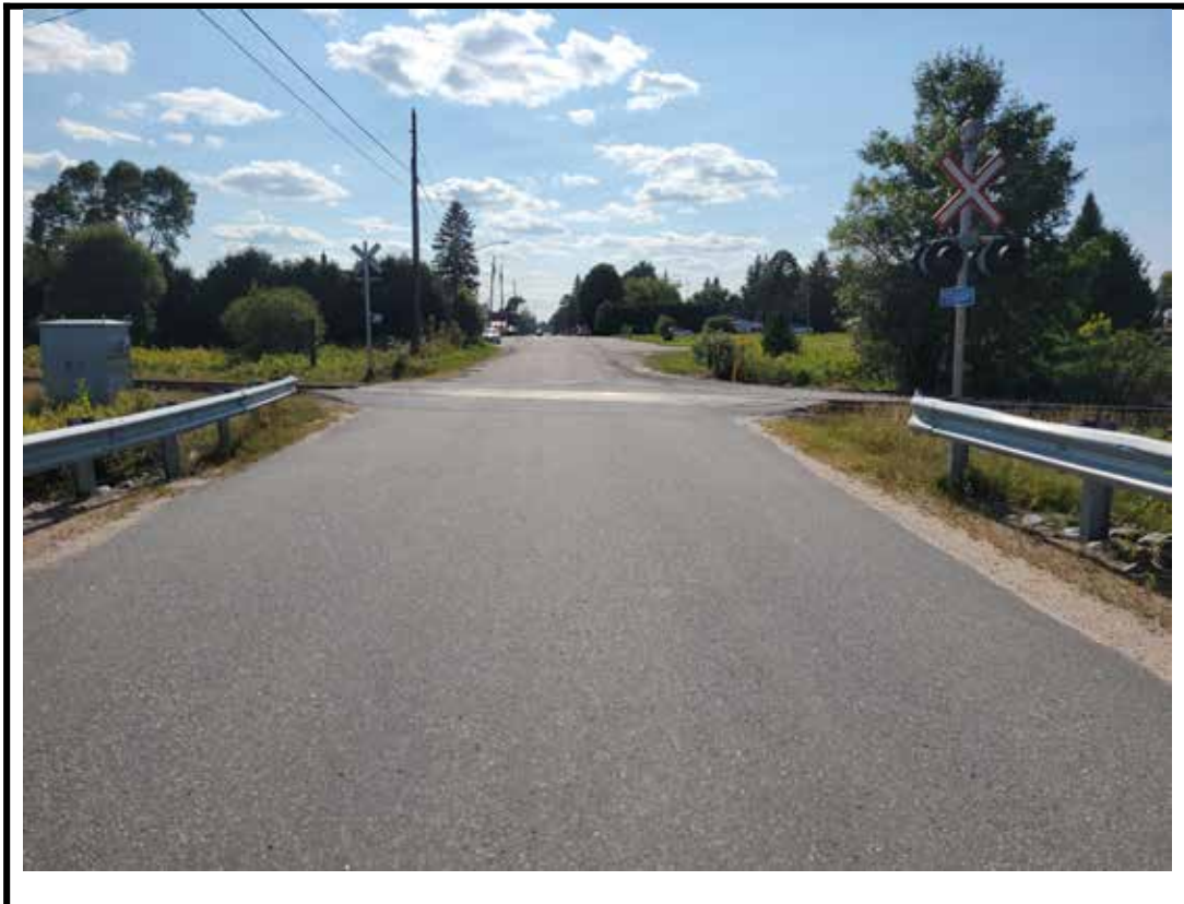
Photo 4 West approach from center of structure
