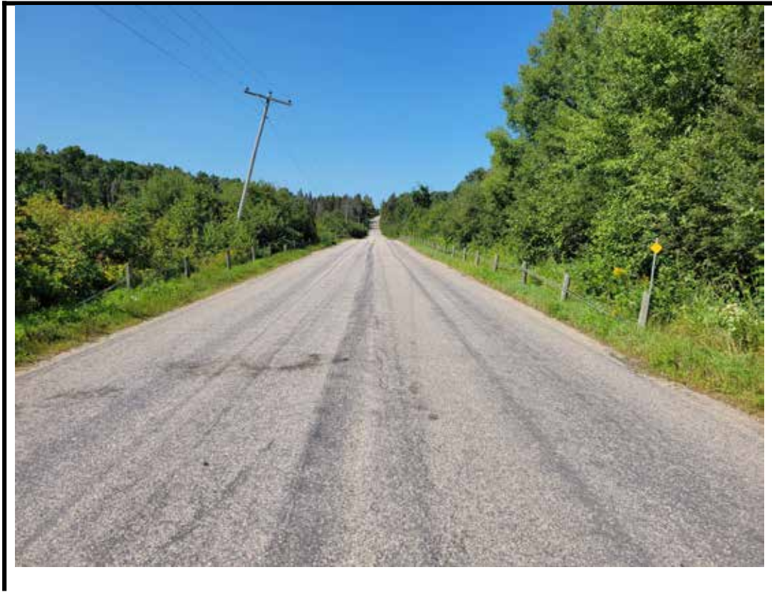
Photo 1 Structure from east approach
