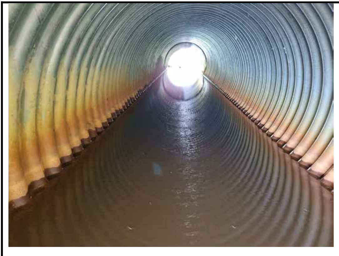
Photo 8 Interior view of culvert barrel
