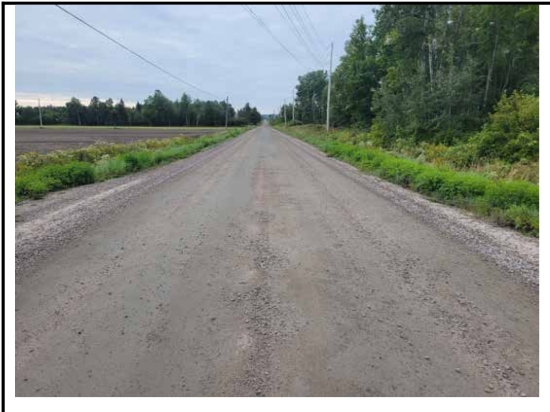
Photo 4 South approach from center of structure
