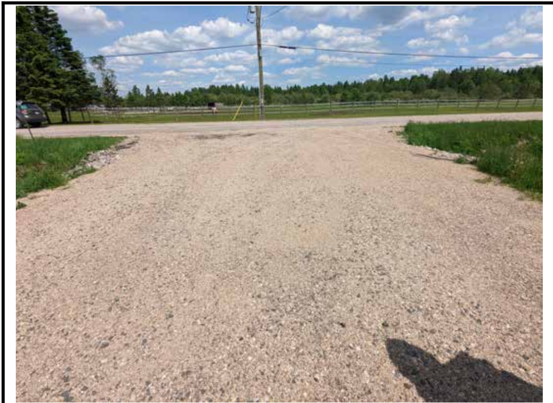
Photo 2 Structure from West approach
