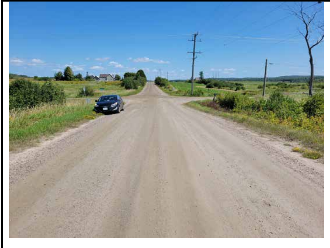
Photo 3 East approach from center of structure
