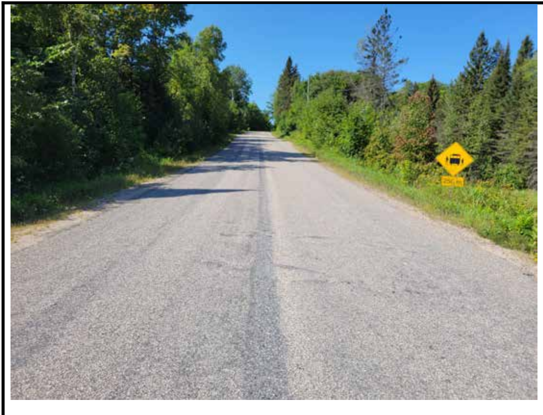
Photo 4 West approach from center of structure
