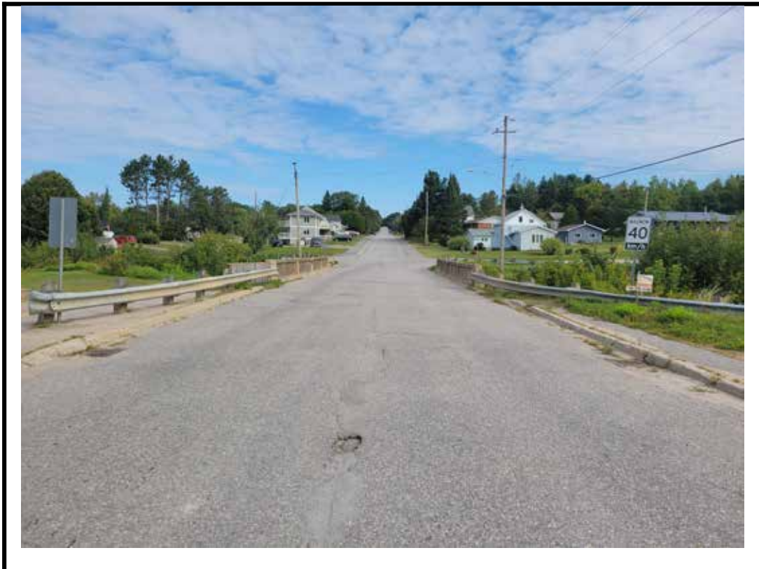
Photo 2 Structure from south approach
