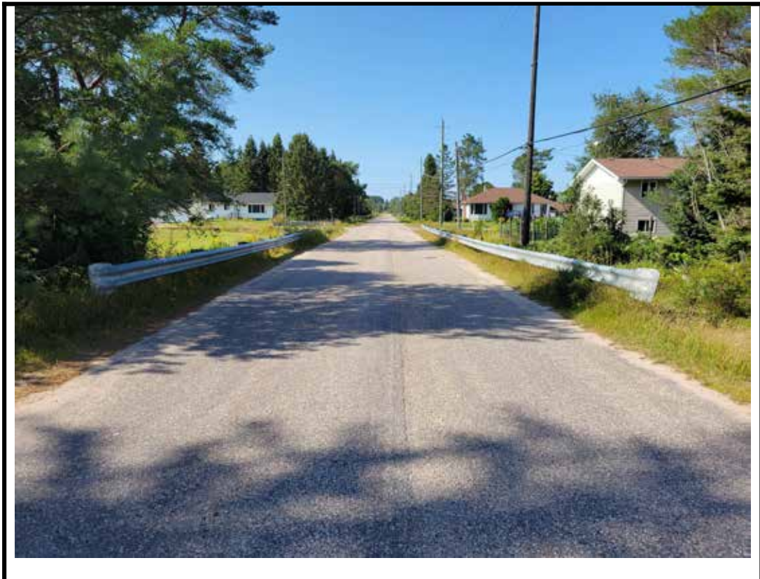
Photo 2 Structure from south approach
