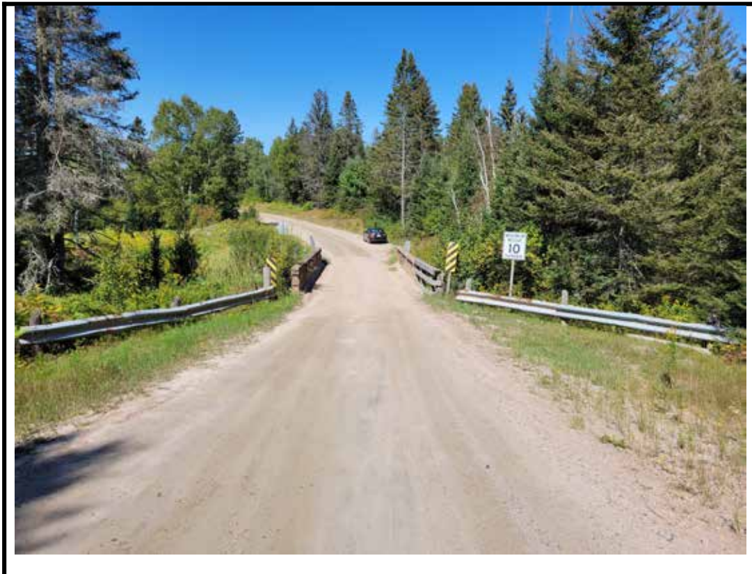
Photo 2 Structure from south approach
