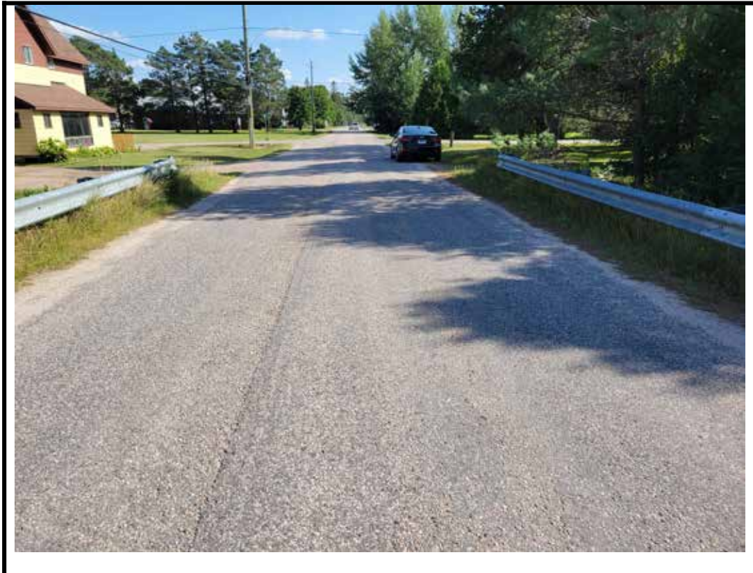
Photo 4 South approach from center of structure
