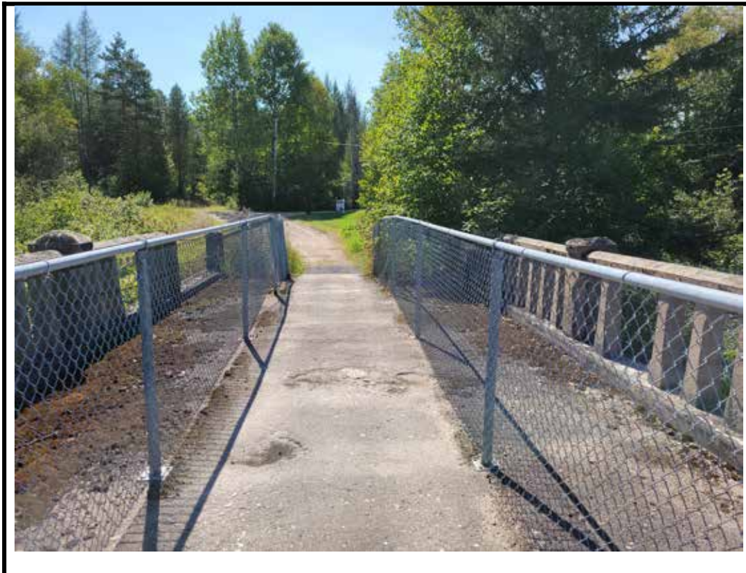
Photo 4 West approach from center of structure
