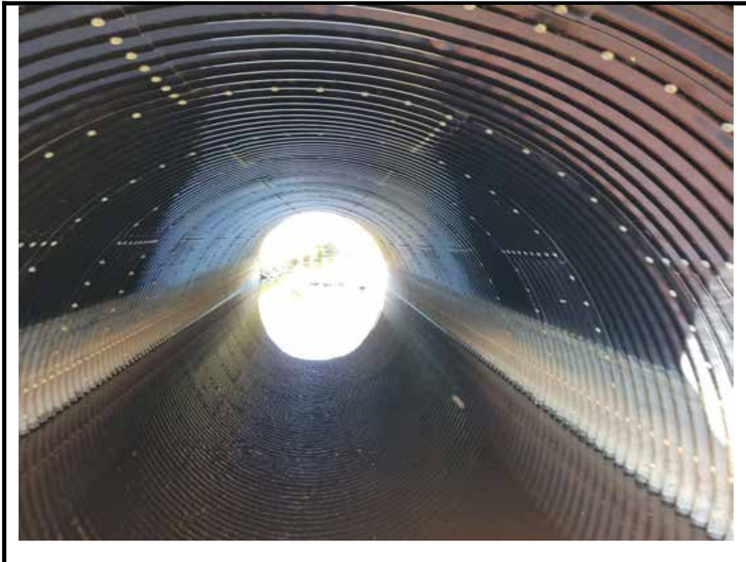
Photo 10 Interior of culvert barrel
