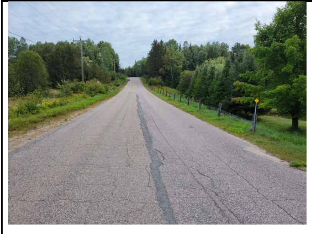
Photo 2 Structure from south approach
