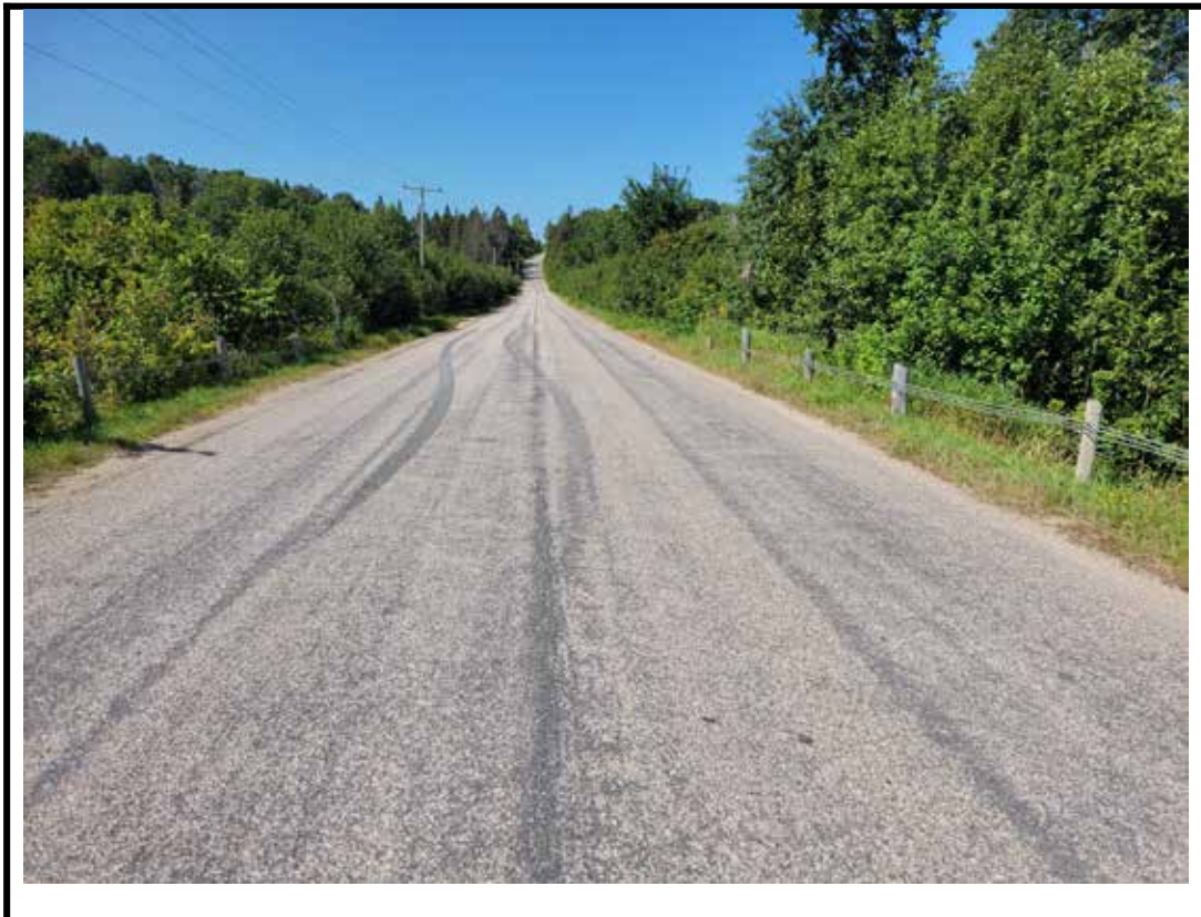
Photo 4 West approach from center of structure
