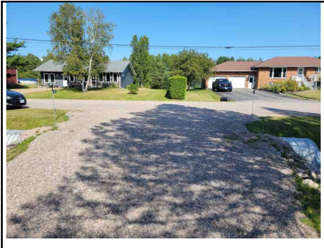
Photo 2 Structure from West approach
