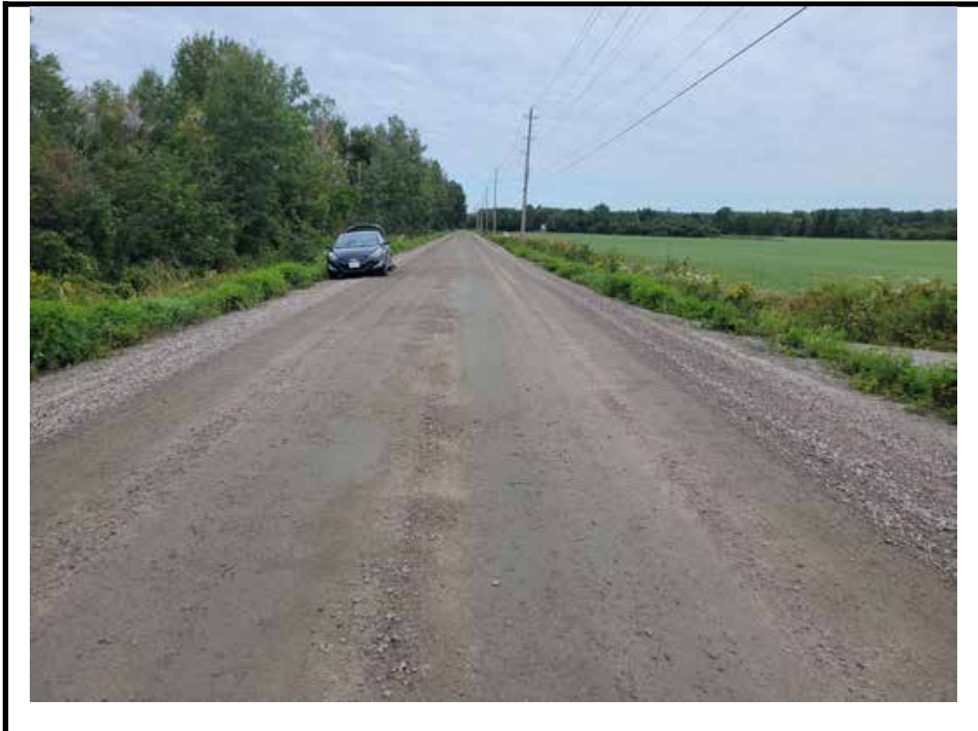
Photo 3 North approach from center of structure
