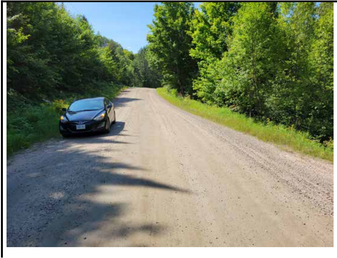
Photo 3 North approach from center of structure
