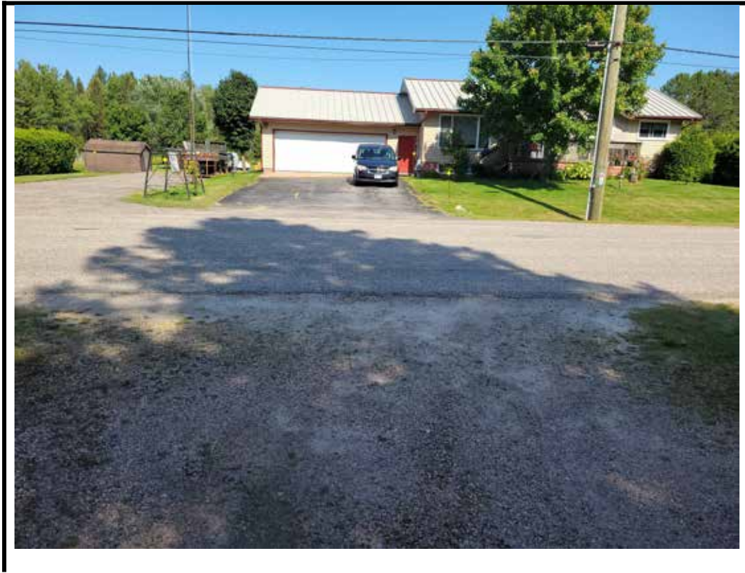
Photo 3 East approach from the center of structure
