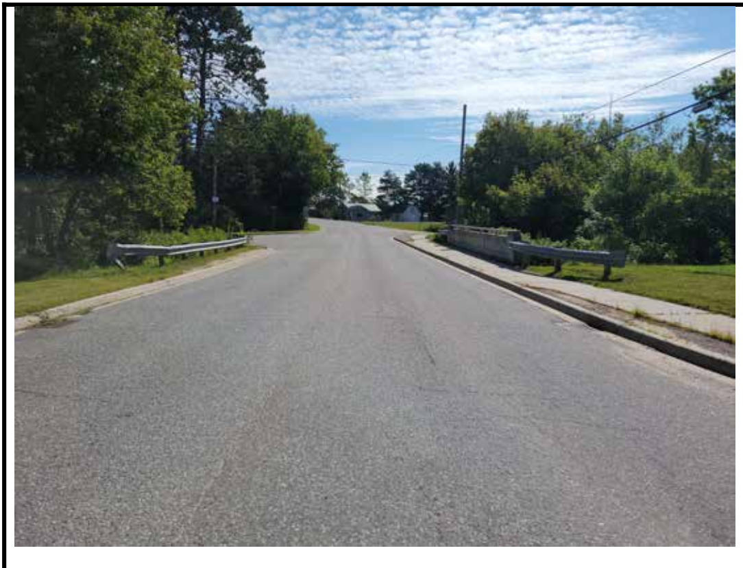
Photo 2 Structure from west approach
