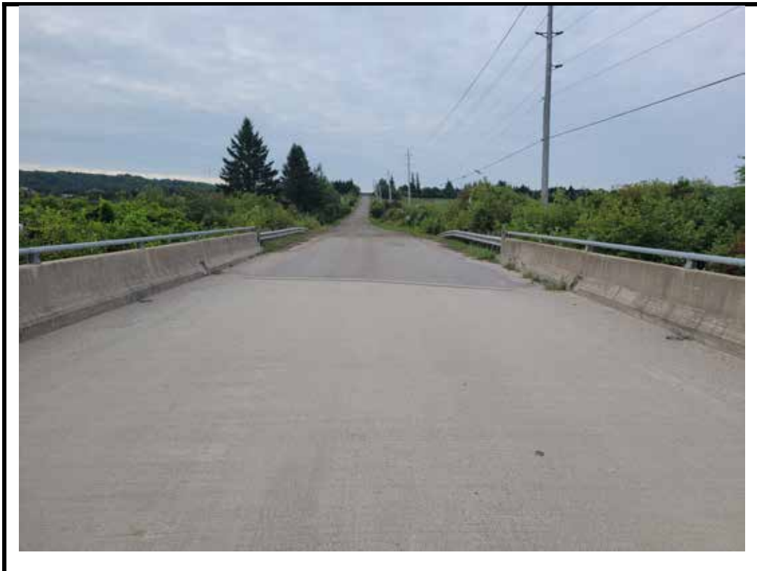
Photo 4 South approach from center of structure
