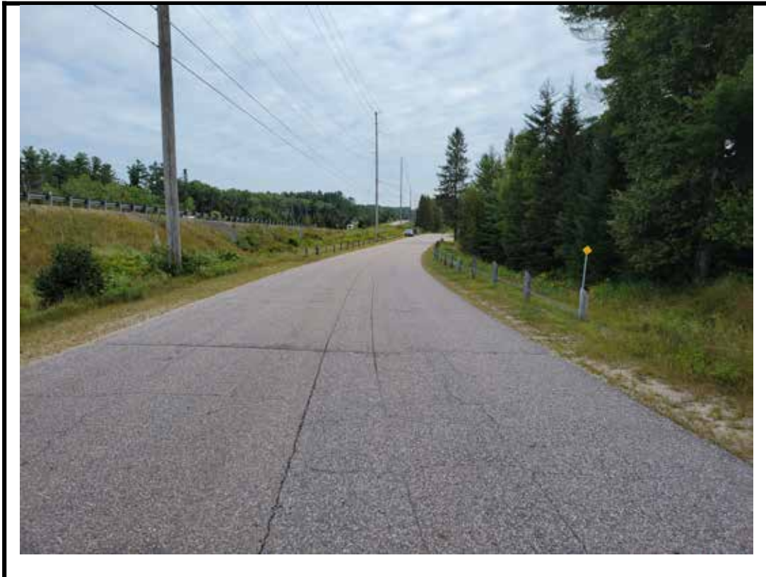
Photo 2 Structure from south approach
