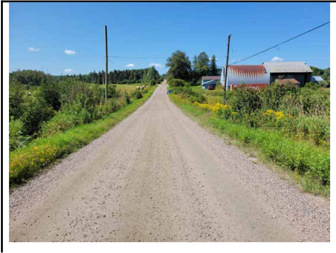
Photo 1 Structure from east approach
