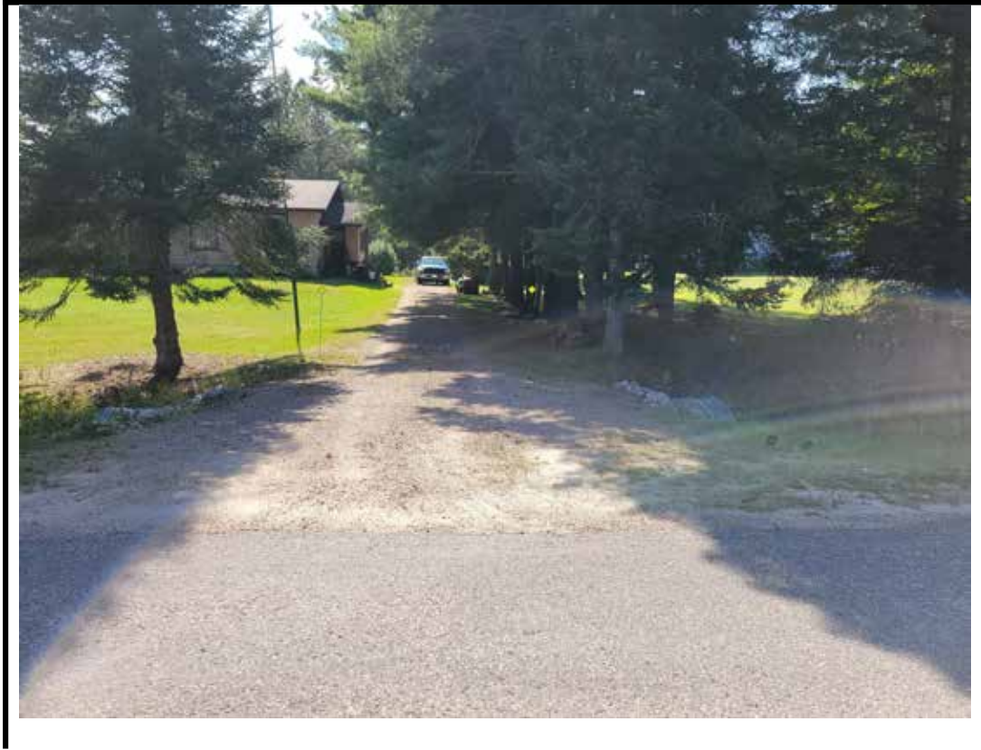
Photo 1 Structure from East approach
