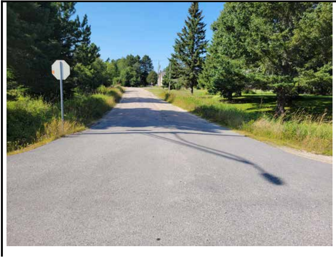
Photo 3 North approach from center of structure
