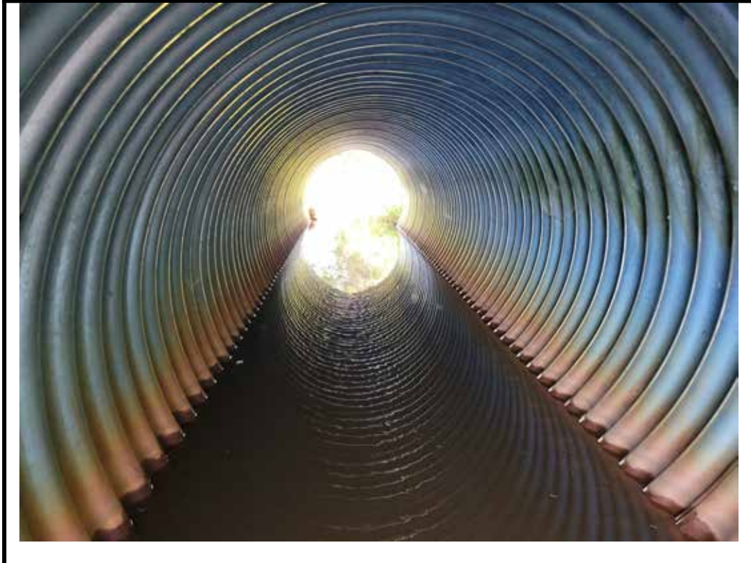
Photo 8 Interior of culvert barrel
