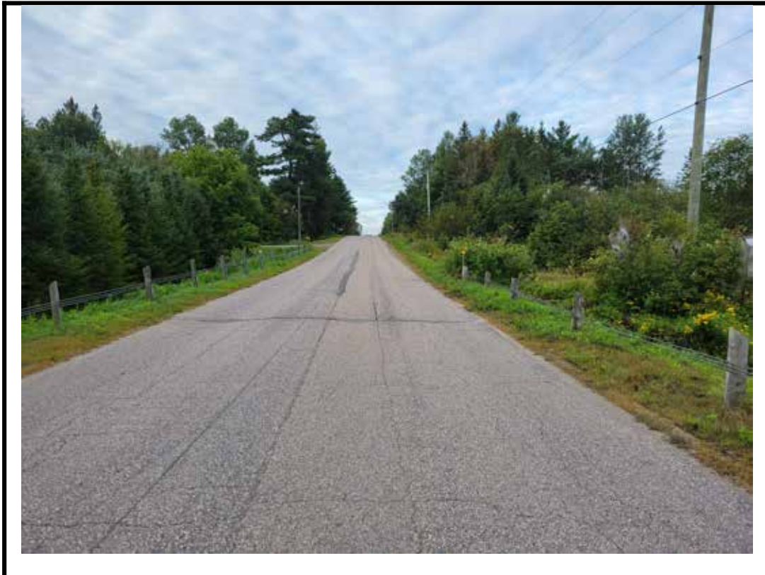
Photo 4 South approach from center of structure
