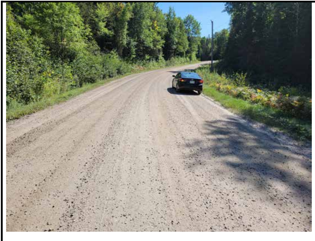
Photo 4 South approach from center of structure
