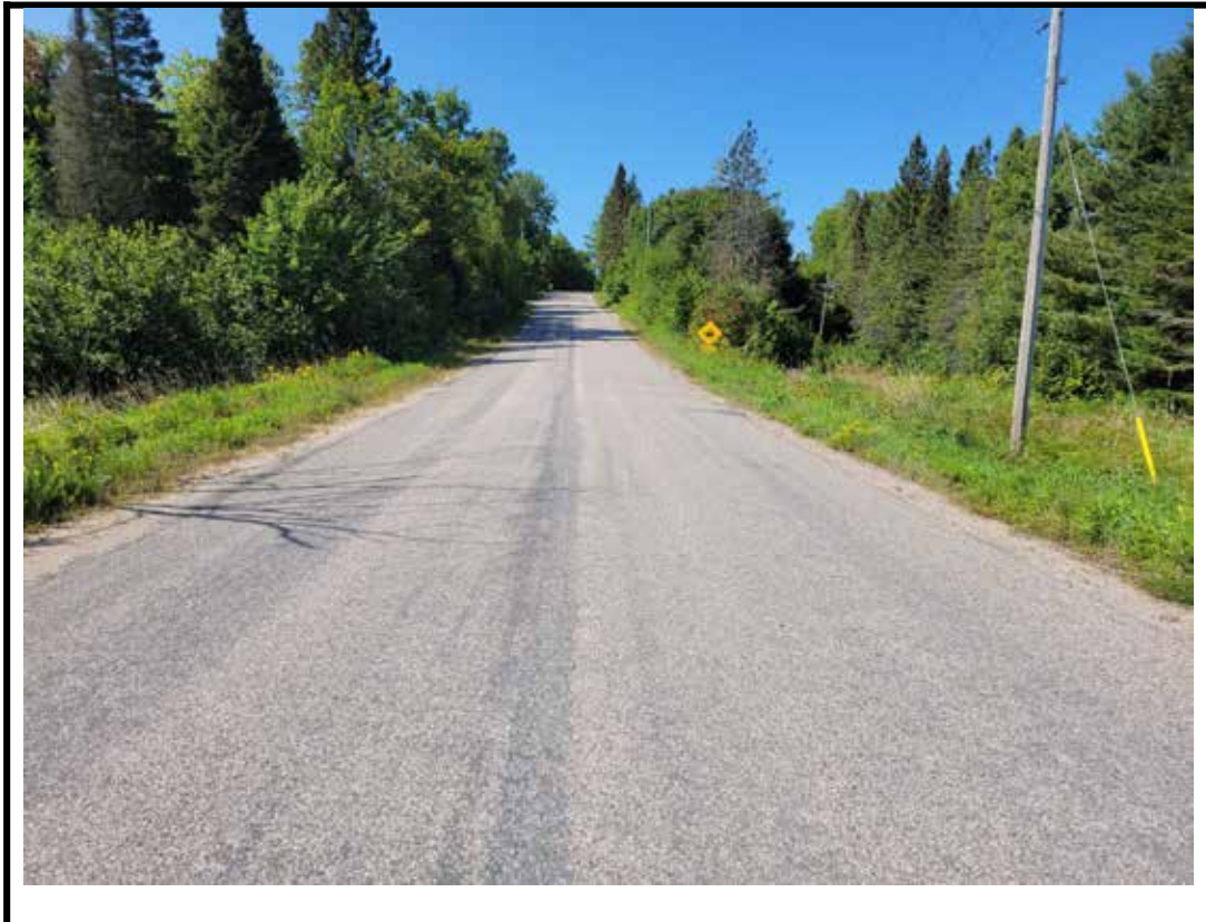
Photo 1 Structure from east approach
