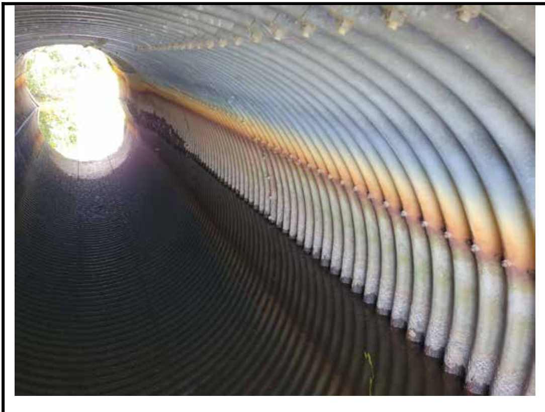
Photo 8 Interior of culvert barrel
