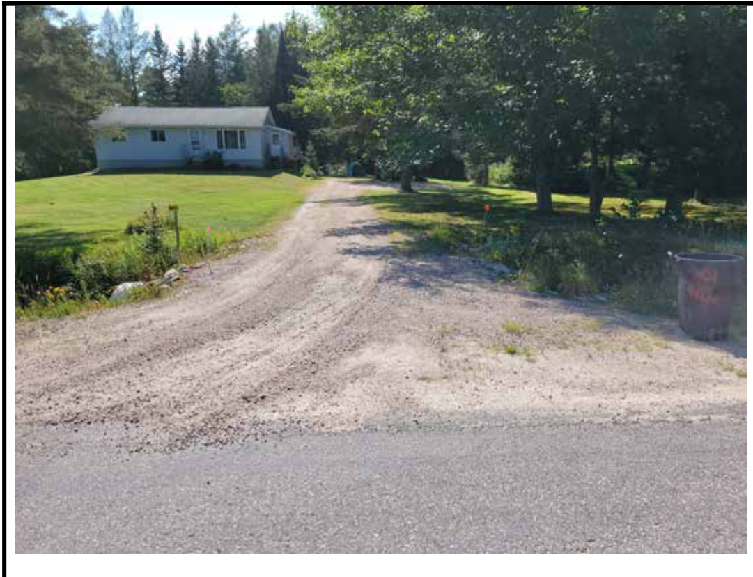
Photo 1 Structure from East approach
