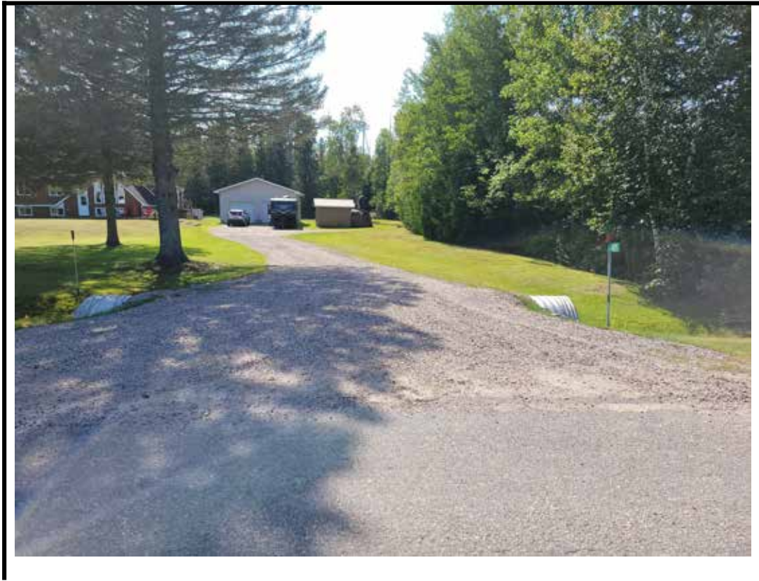
Photo 1 Structure from East approach
