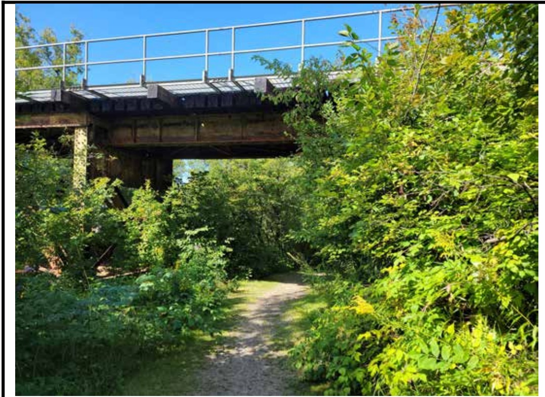
Photo 13 East elevation of north span
