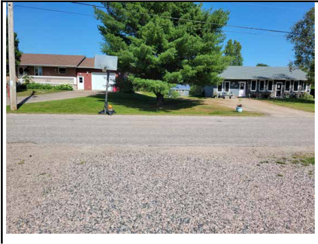
Photo 3 East approach from the center of structure
