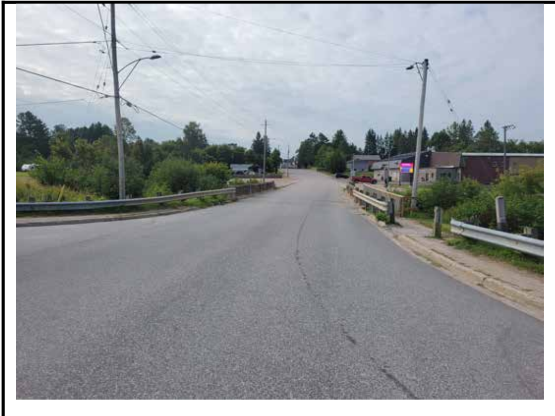
Photo 1 Structure from north approach
