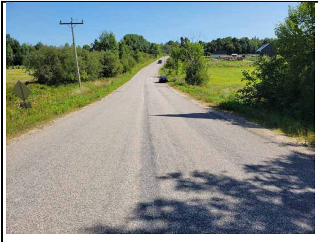
Photo 2 Structure from west approach
