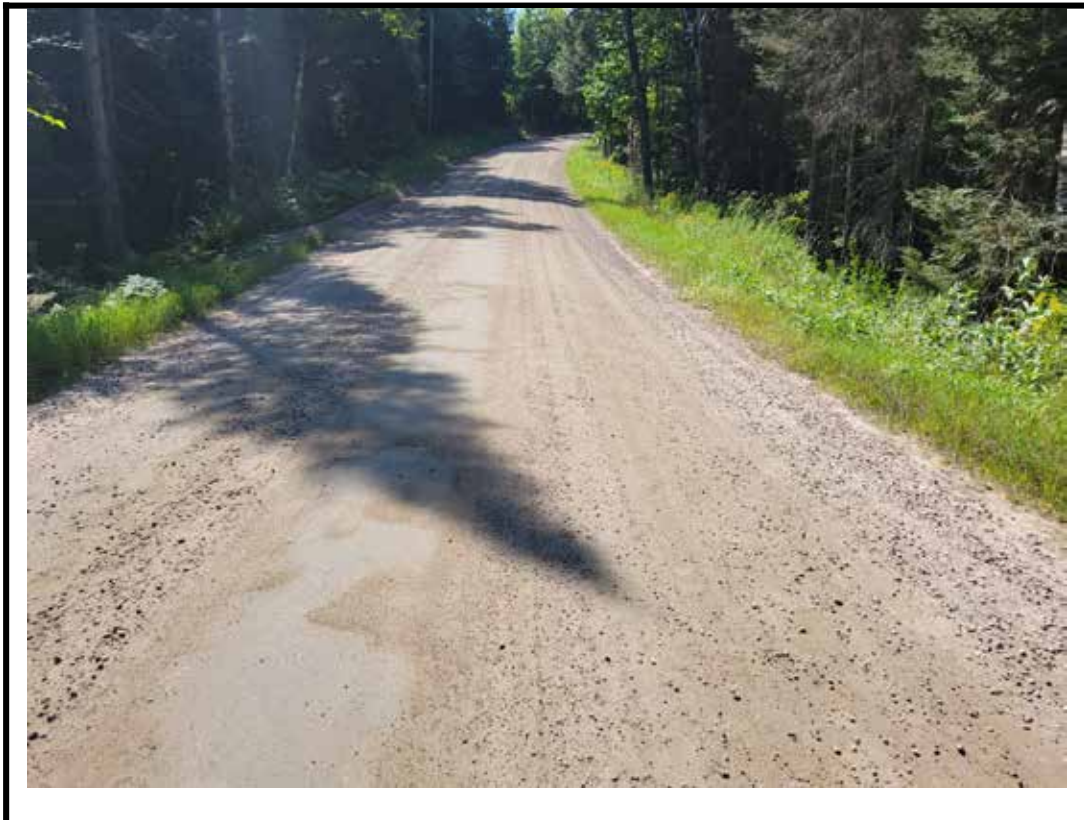
Photo 4 West approach from center of structure
