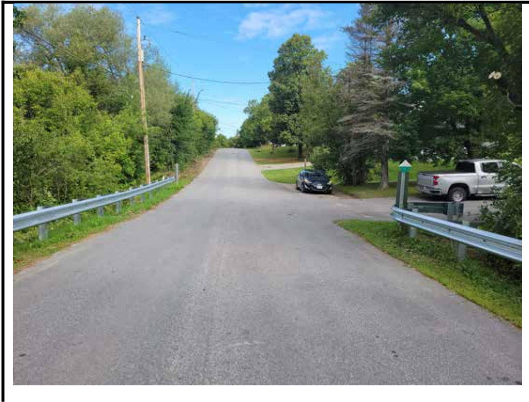
Photo 3 North approach from center of structure
