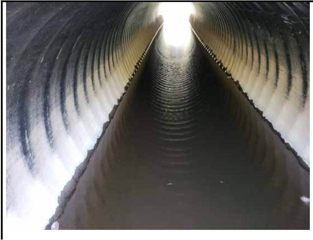
Photo 7 Interior of east barrel; replaced since 2022 inspection
