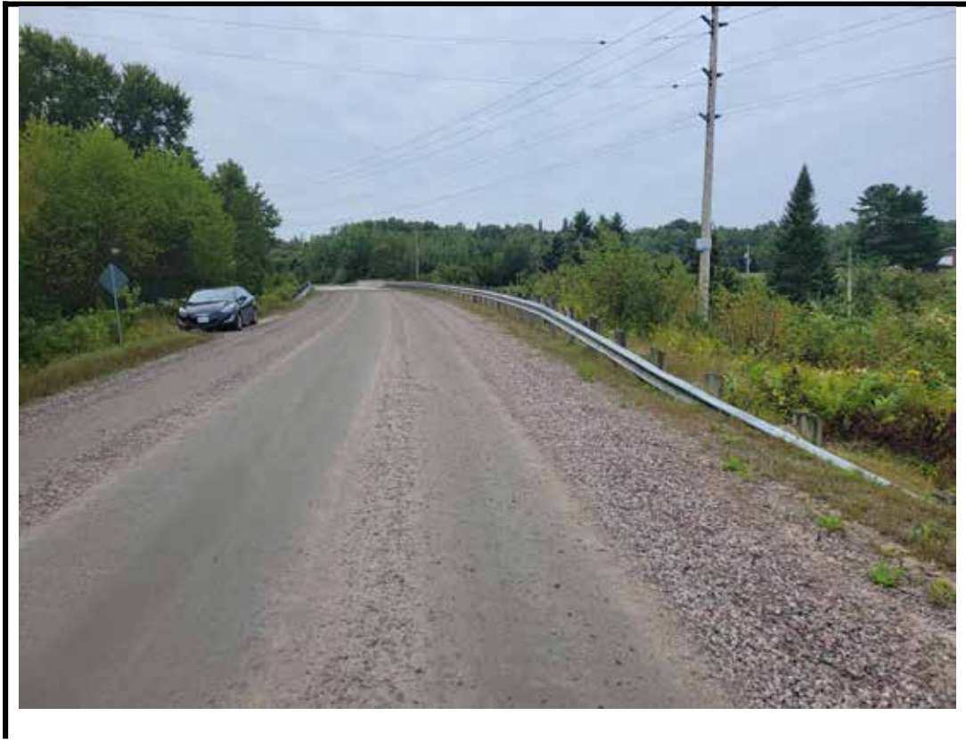
Photo 1 Structure from north approach
