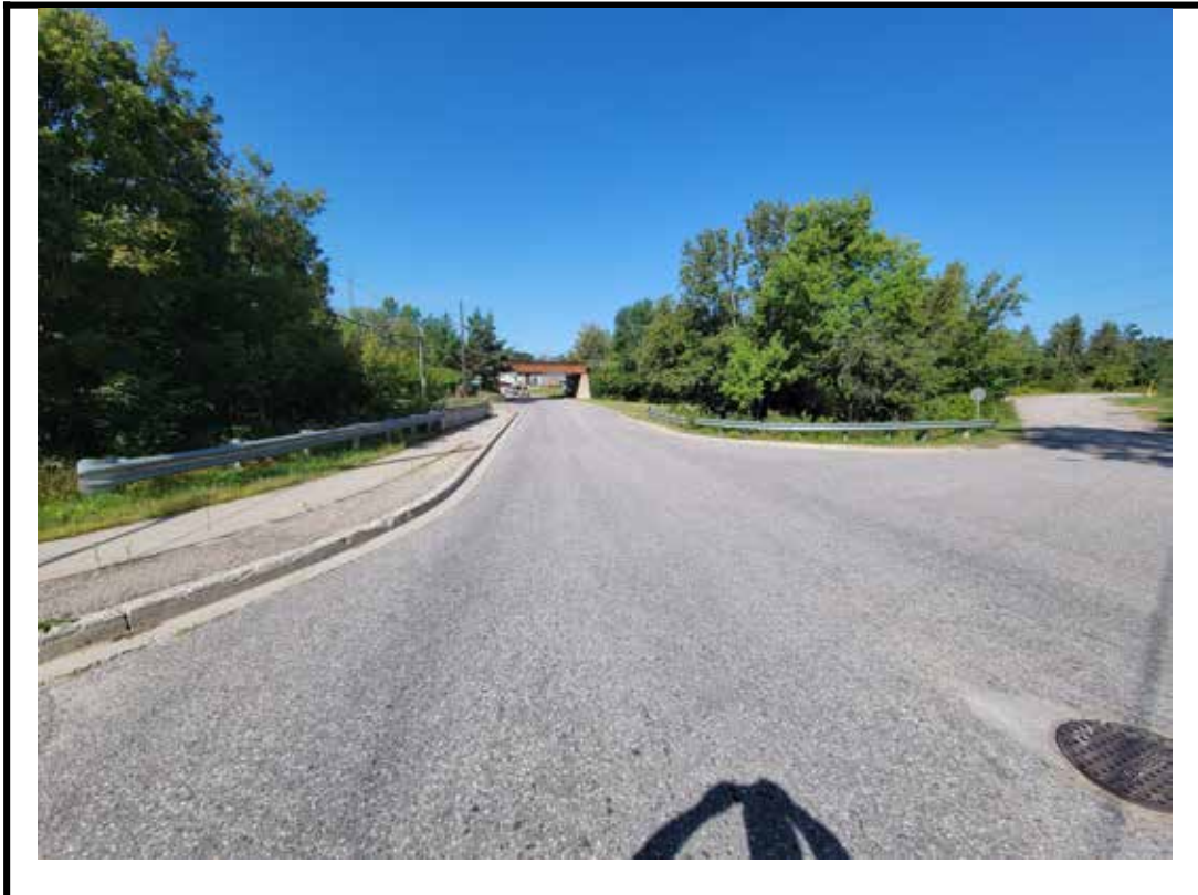
Photo 1 Structure from east approach
