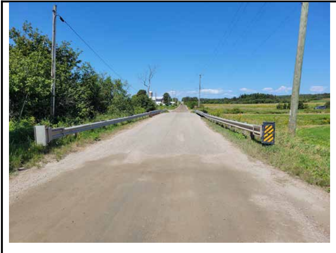
Photo 2 Structure from south approach
