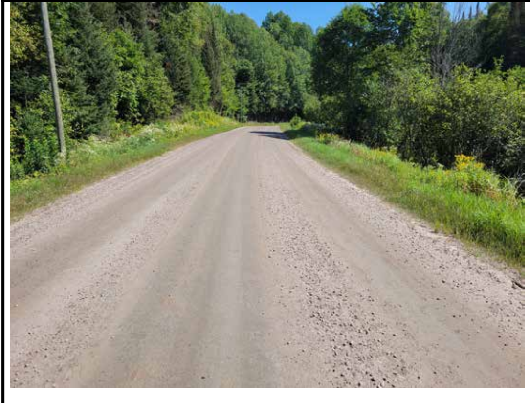
Photo 2 Structure from west approach
