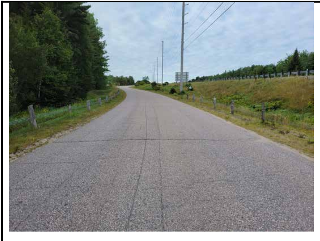
Photo 4 South approach from center of structure
