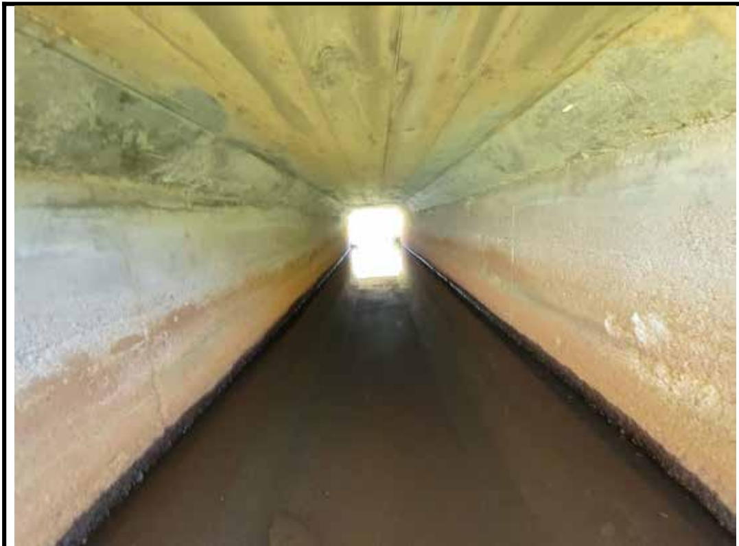
Photo 8 Interior of culvert barrel
