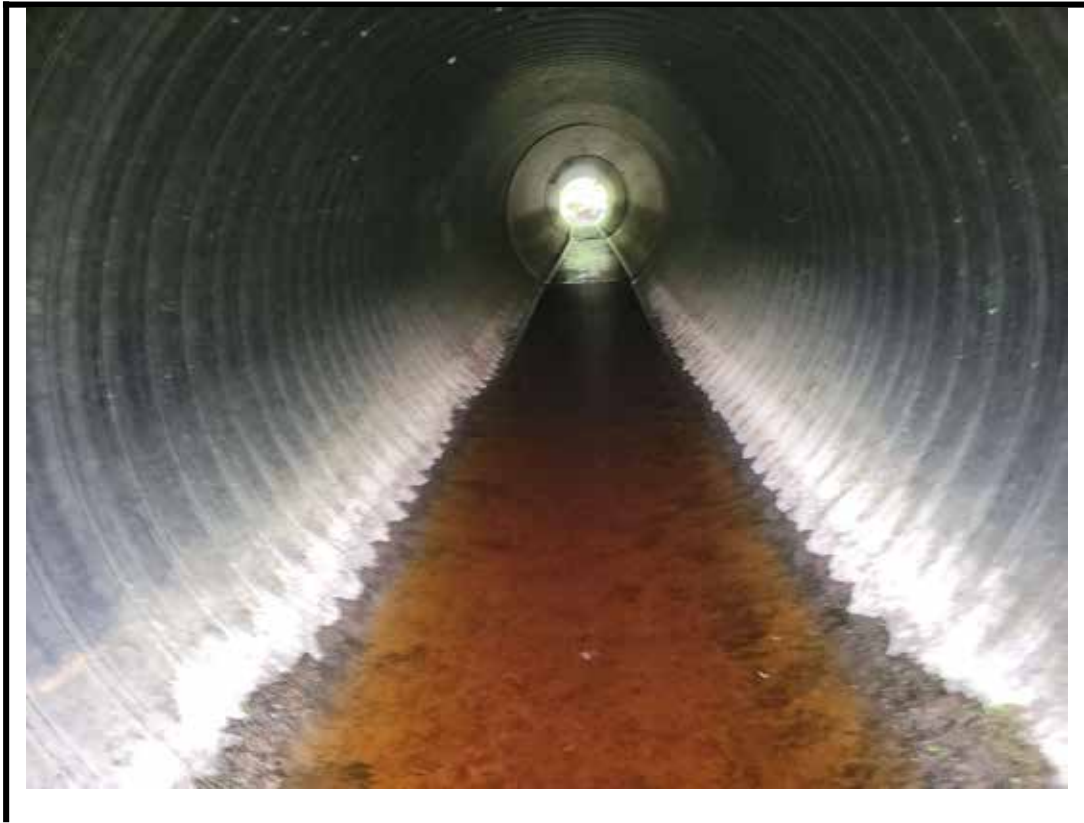
Photo 7 Interior of culvert barrel
