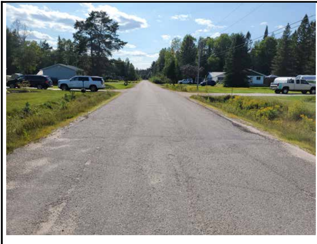
Photo 4 West approach from center of structure
